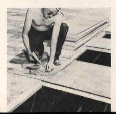
· A new type of fire-retardent roof construction has been developed to improve the fire resistant qualities of industrial roofs. Lexsuco roof is designed to (1) prevent dripping of inflammable asphalt or tar, (2) eliminate all combustible materials between roof deck and insulation and (3) improve roof rigidity, thus minimizing buckling of the steel roof deck during a fire.
