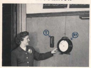
Miss K. Mart, Teacher in Room 14 Lincoln School, Racine, Wis. "T" is POWERS Type A Thermostat installed in 1903. It controls mixing dampers. Thermostat was set for 75° F. Note even control during schools hours. "RT" is Recording Thermometer which made charts at right in February 1953.
