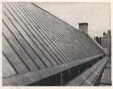
10,000 LBS. OF REVERE SHEET COPPER were used for the standing seam roof, valleys, gutters and base flashing. Note expansion joints in gutters 32 feet apart.
