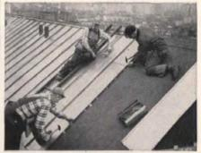
PREFABRICATED PANS of 16 oz. Revere Copper being fastened into place with cleats, using two nails per cleat. Pans are 1714" wide by 8' long and attached top and bottom with loose lock cross seams.
