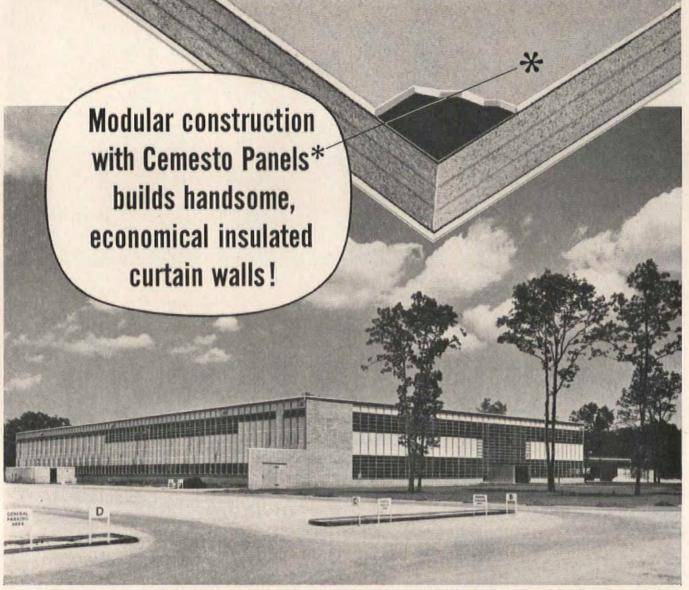
Stratas Division Plant of Fairchild Engine & Airplane Corp. at Bay Shore, L. I., N. Y., shows its handsome Cemesto Panelized exterior. Here is a unique combination of striking modular design plus functional use of panel materials.
