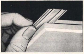
Aluminum spline is inserted in kerfed edge of Fiberglas Acoustical Tile, 24" x 24" x <sup>3</sup>/<sub>4</sub>".
