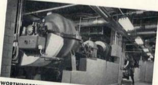
WORTHINGTON'S DESIGN for these two 625-ton centrifugal refrigerating units called for special finned aluminum tubes
