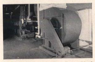
Air for drafting rooms and modeling studios is conditioned by 24 specially built, automatically controlled American Blower Air-Conditioning Units. Each unit contains heating and cooling coils and capillary air washers.
