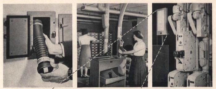
Typical installation of the Automatic Selective Pneumatic Tube System. Left: Tube carrier being placed in a transmitting tube. Center: The medical records room where employees are on hand around the clock. Mis-directed carriers come to this point for return to the sender. *Right:* Central control station. Signal panel is at left center. Systems of this type are in operation at Johns Hopkins Hospital, Baltimore, Md., and Genesee Hospital, Rochester, N. Y.
