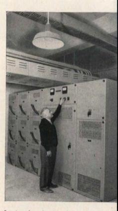
Low-impedance bus duct riser carries power from low-voltage switchgear to panelboards, located in wire closets on each floor.
