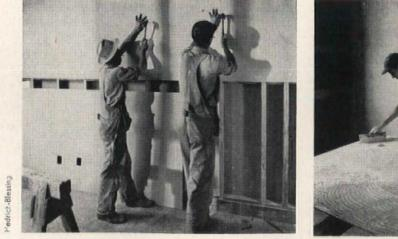
Crew nailing first layer of gypsum wallboard to wood studs. Layers are each  $\frac{1}{26}$  in thick
