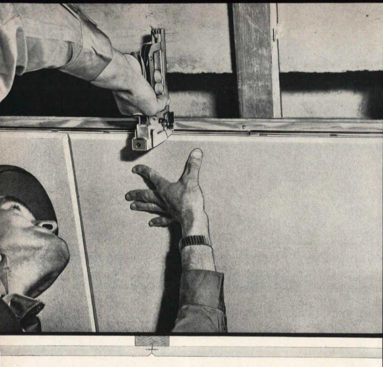
If you've ever been bound by a budget limited to ordinary tile nailed or screwed to wood furring, this is important news for you. It's the "Ful-Spline" System for Fiberglas tile the installation method that makes Fiberglas Acoustical Tile your *lowest cost non-combustible ceiling!*
