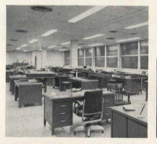
General offices, private offices and conference room are lighted by 854 runs of 8-ft. Day-Brite Low-Brightness Lens troffers recessed into a modern grid type suspended ceiling. Equipped with Holophane Controlens\* to reduce glare, these fixtures furnish extremely comfortable illumination. \*®HOLOPHANE CO., INC.
