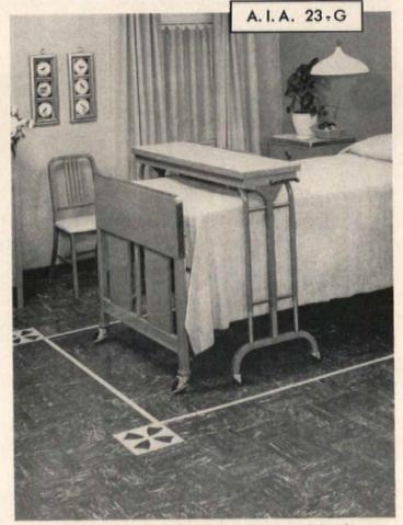
KENRUBBER TILE FLOORS can be planned and designed to fill any decorative or functional need. For instance, the ThemeTile and Feature Strip shown in a private room here can easily and economically be installed in wards and corridors for directional lines, traffic lanes and area demarcations.
