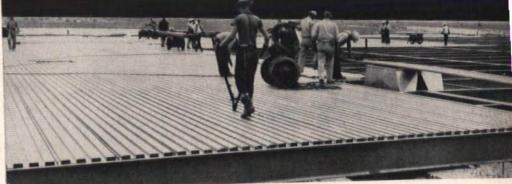
The many unique features of Robertson Q-Deck make it of special interest to the architect and engineer who is concerned about the fire hazard aspect of his flat roof design. To begin with, Robertson Q-Deck is designed with tight side and end laps to eliminate the need for an inflammable vapor seal. Its two-foot width and long span characteristics mean fewer joints, and its zinc-coated surface (or basic Galbestos) eliminates the need for field painting.
