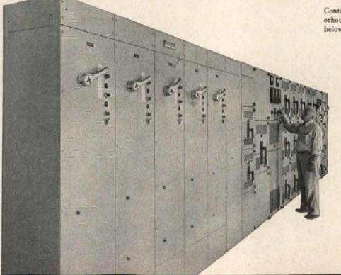
Control Center Balcony Location in the powerhouse allows the operator to see the motor, below, while inspecting its control unit.
