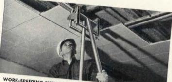
WORK-SPEEDING METHODS, such as this new way of crimping aluminum ceiling panels to water-circulating aluminum tubing resulted
