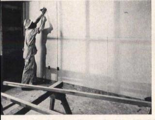
Temporary nailing of face layer. Minimum nailing holds panel until adhesive develops adequate bond
