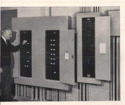
Tripped circuits can be seen at a glance—because all Westinghouse De-ion Circuit Breaker handles assume central position on automatic tripping.
