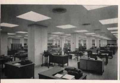
Mistakes are held to a minimum in the company's Underwriting Department. Here, the distracting clatter of typewriters, business machines, and voices is effectively muffled by the Arrestone ceiling. This material offers a maximum of sound absorption.
