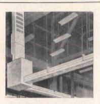
Type LVD Flex-A-Power feeder busway connecting with type FVK Flex-A-Power take-off which provides power outlets at one foot intervals. Both available with either copper or aluminum bus bars.
