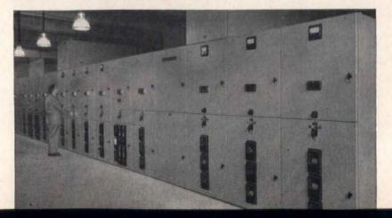
MAIN HIGH-VOLTAGE SWITCHGEAR feeds and protects 19 spot networks throughout the 15-building research center.
