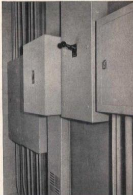
Panelboards are mounted in wire closets on each floor. They provide for centralized control of electrical services.
