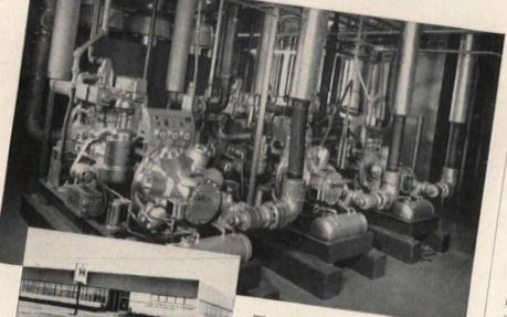
This 100-ton capacity Ready-Power in-stallation air conditions the Interna-tional Harvester Parts Depot, Dallas.
