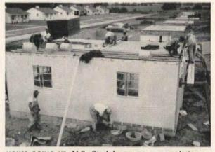
HOUSE GOING UP. U.S. Steel home nears completion as workmen on scaffold (right) bolt on exterior panels. These sturdy homes offer quality construction at budget price.
