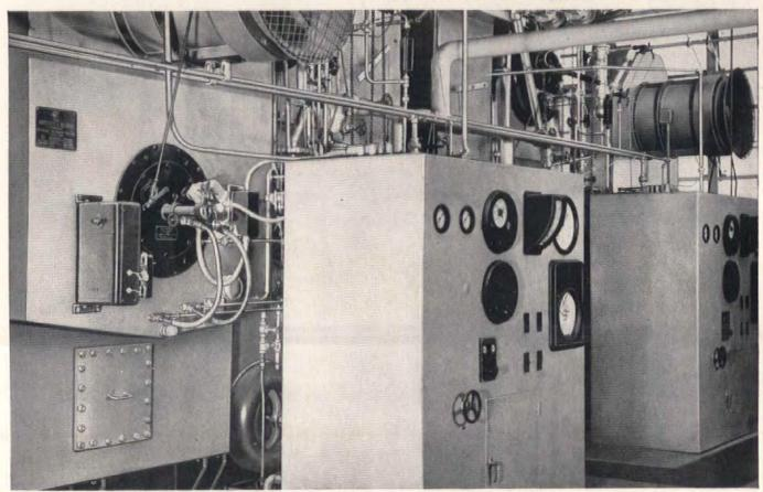
These two Type FM, B&W Integral-Furnace Boilers supply steam for all heating, cooking, and laundry requirements at a large midwestern hospital.
