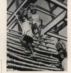
Scaffolding in Asia is most often made of strong and flexible bamboo, but is very seldom crossbraced. Workers must cling to the bamboo with their fingers and toes, for the scaffoldings are not usually equipped with foot-boards
