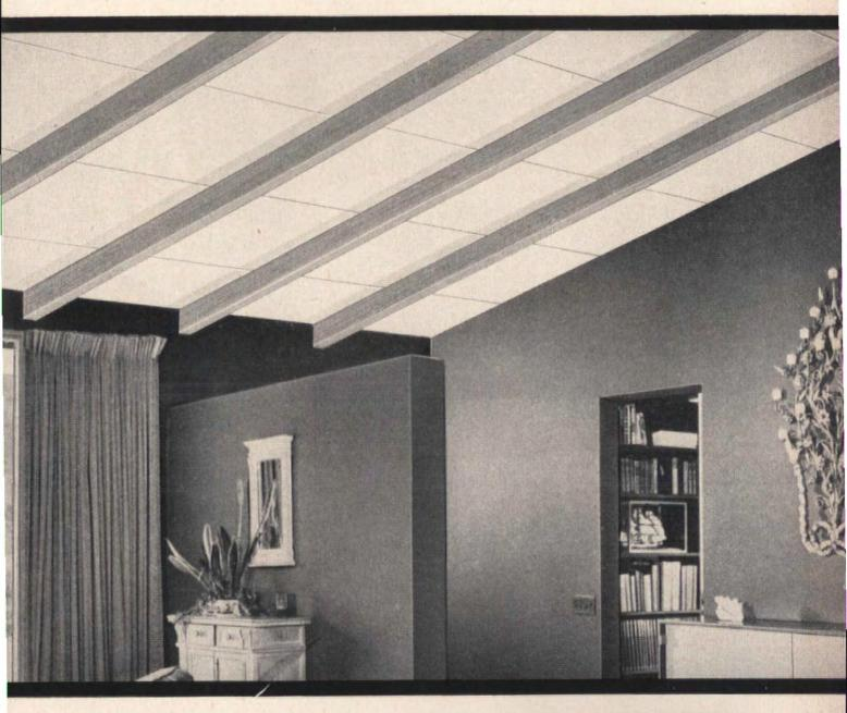
The secret's in the seal! Exclusive vapor barrier lets you build exposed beam ceilings for less, anywhere in the U.S.A. Continuous vapor barrier combines (1) a membrane laminated into each unit, plus (2) a rubber gasket that seals carefully machined T&G joints. Protects against condensation within the deck in any climate. (Also available without vapor barrier for use in moderate climates.)
