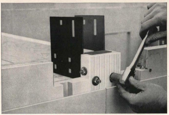
RAISING THE ROOF of a U.S. Steel home goes faster with help of RB&W bolts. Here workman is tightening bolt holding steel plate to exterior wall panel. Plate is then used as joint for bolting ceiling panels.
