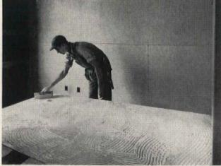
Spreading adhesive over back of face layer, which will be applied in vertical strips over first layer
