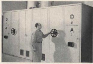
**DEPENDABLE CONTROL** for motors driving Carrier corpressors is provided by this 5000-volt G-E unit, which w ready for operation upon installation.
