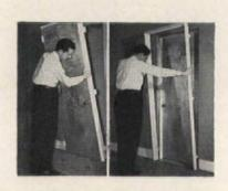
Packaged door needs only screwdriver for installation
