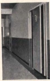
RECESSED IN CORRIDOR WALL, this 71/2ton G-E unit sends conditioned air to surrounding offices. Air returns through louvers in doors to unit.
