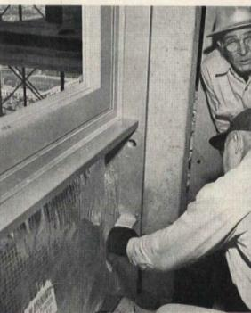
Left, details of wall construction. Panels are ½-in. aluminum backed with 1½-in. of glass fiber and aluminum foil (see also photo above). Note space for high-velocity air ducts between conditioner units; also that overlapping wall panels are virtually self-flashing
