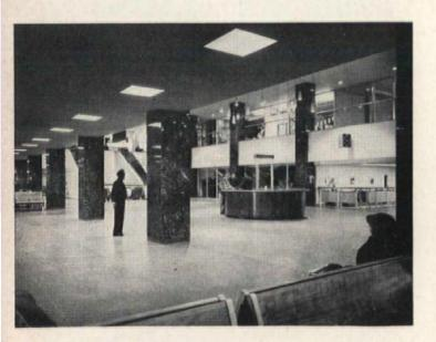
The photos on this page picture the waiting room with its large two-story concourse. This is the area where terminal and commercial building meet. Walls and columns are finished in marble; most of the interior trim and the doors are aluminum; the floor is terrazzo; the ceilings are mineral acoustic tile.
