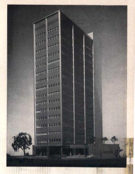
Note exterior columns outside the building skin to simplify office layout, and fact that only two interior columns interrupt clear tower floor space; potential demand for small suites is satisfied by column layout. Building is air conditioned with ceiling ducts which penetrate webs of large girders
