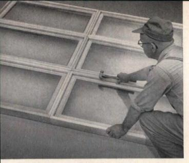
Mr. Hilferding states further that, "Flexivent permits adaption to any type of construction by the use of built-ups and casing." In building up Flexivent group, workman makes certain that units are kept square and properly aligned. This is important.
