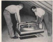
Easily installed — Simply place the Hunter Attic Fan over ceiling opening on attic floor or joists. Modern automatic ceiling shutter with metal trim screw-fastens from below.
