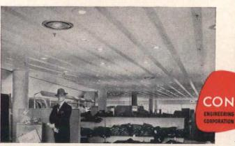
HUTZLER'S, Towson, Md. (above), uses special Kno-Draft High Pressure Air Diffusers that permit the air supply in a given area to be changed without unbalancing the air delivery of the other outlets, or creating objectionable noise. Installed cost comparable to conventional system.
