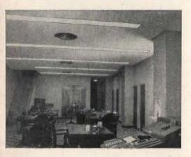
Recessed lighting and air-conditioning fixtures are readily installed with a Travertone ceiling. In the vault area, Travertone prevents the sounds of business machines from building up to disturbing levels.
