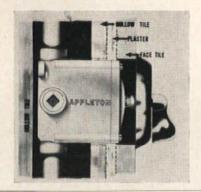
line connection purposes, and line wires are spliced in the *Unilet* body. This factory seal eliminates the need for sealing fittings normally required within 18 in. of arcing devices as specified in Article 500 of the National Electrical Code.
