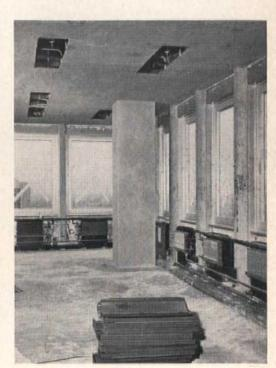
Above, further steps in erecting curtain walls: 1, positioning and bolting panel through holes cast in mullions; 2, vertical joints; 3, windowless portions ready for insulating, lightweight concrete backing; 4, wall panels up, conditioners in, acoustic ceiling and recessed fluorescent fixtures installed. Below: only at four corners of panels was flashing needed
