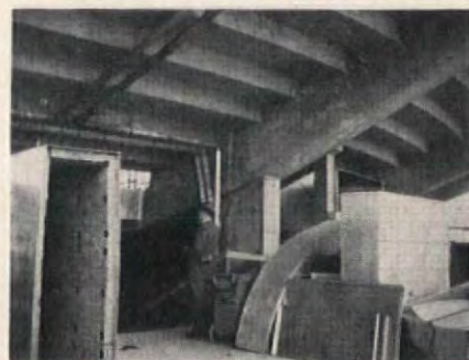
Above: inside auditorium peering through scaffolding toward podium. Below: stepped level of auditorium floor cantilevers toward lobby on girders to be partly exposed
