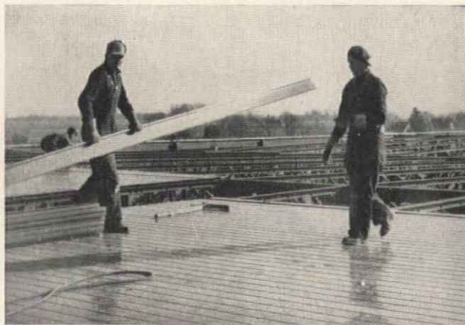
FERROBORD® STEELDECK provides interlocking units long enough to span three or more purlins. No scaffolding needed for erection; work is done from above. Can be clipped or welded to joist. Write Truscon for facts.
