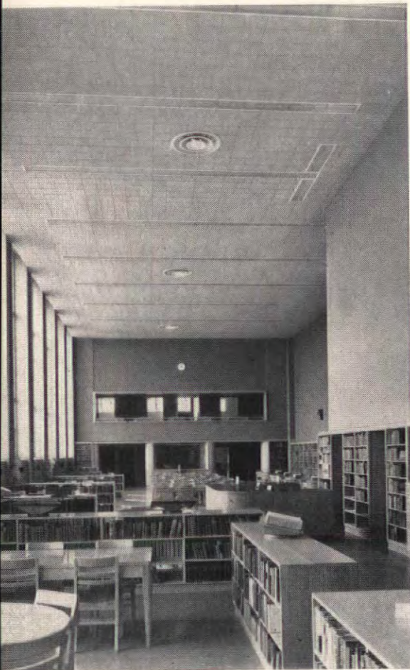
Undisturbed quiet in the library is essential to concentration. This quiet is assured by the Cushiontone ceiling. Easily nailed or cemented in place, Cushiontone does not interfere with the installation of recessed lighting and air conditioning.
