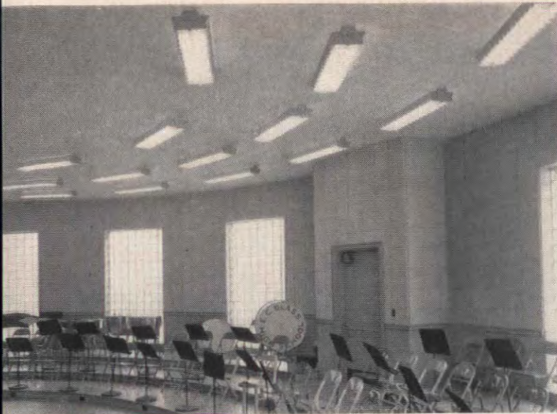
the band room, sound-absorbing Cushiontone covers the ceiling and upper walls. This acoustical treatment helps prevent build-up of distracting noise levels and provides proper acoustics.
