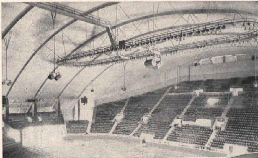
Flood and spotlights for general and special lighting of the new State of Alabama Agricultural Coliseum are mounted on a catwalk 76 feet above the arena floor with a connected load of 222 Kw. Transformers and feeder panels are on the ground. ELECTRUNIT E.M.T. was used for both installations.
