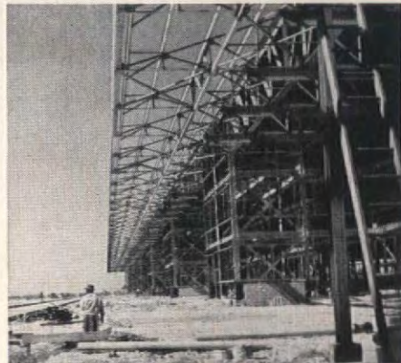
View of steelwork for 1219-foot-long hangar.
