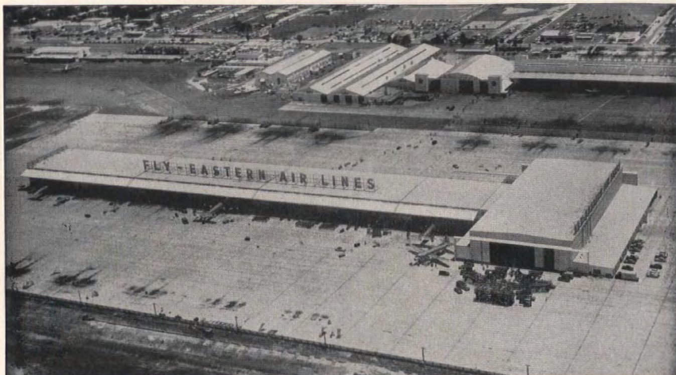
Aerial view of Eastern Air Lines' base at Miami International Airport. Maintenance building in foreground designed by Leslie B. Taylor, consulting structural engineer, of Miami. Construction supervised by J. Herbert Shurtle, Eastern Air Lines engineer. Steelwork fabricated and erected by Bethlehem Steel Company.
