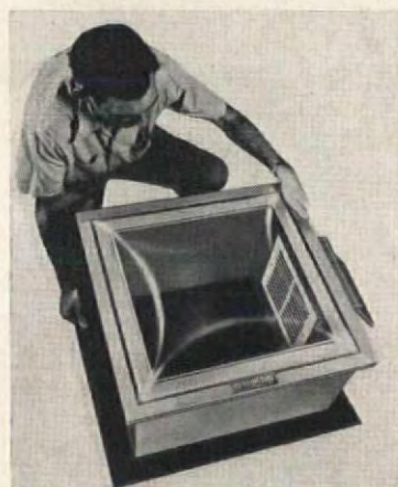
Looking through clear plastic dome of vent shows air-intake louver
