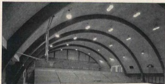
High school gymnasium, size 190x168 feet, with seating capacity of 4,500. Roof is supported by glued laminated timber arches spaced at 19 feet. Roof deck is two-inch tongue-and-groove sheathing with built-up surface. Architect: Donald W. Edmundson, Portland, Oregon.
