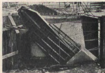
Above: a closeup of the dome casting which rides on buttress casting like a ball and socket joint. Below: buttress casting, later to be concreted
