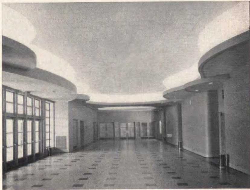
Easily washed or repainted, Cushiontone ceilings in the corridors are simple to keep clean and new looking. A perforated, white painted fiber tile material, Cushiontone soaks up noise efficiently, economically.
