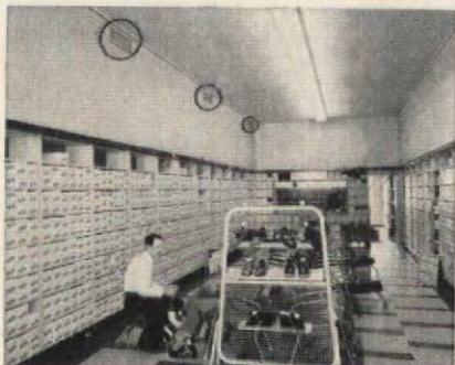
One of 25 stores in Cherrywood Shopping Center (shown in aerial photo) Wantagh, L. I. Warm air delivery registers are circled in photo above.
