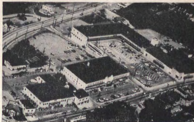
Brentwood-Whitehall Shopping Center built on two levels has 25 shops in 210,000 square feet—80% are air conditioned—parks 1,000 cars. All floors reinforced with Steeltex. Forsyth & Blezard, Architects. Leland Cook, Structural Engineer. Landau Bros., Contractors.
