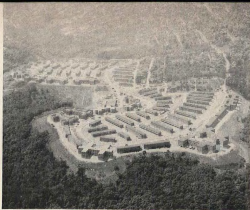
$13-million low rent public housing project, St. Clair Village , 79 buildings, 723 units in 3-story buildings, 366 units in 2-story row houses. Concrete floors poured over Steeltex. Marks, Fisher & Simboli, Architects. George Levinson, Design Engineer. Ragnar Benson, Inc., Contractors.
