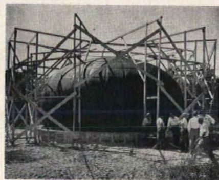
Above: one of the finished bubble houses, ready for occupancy. Below: the inflated balloon, prior to being wrapped in wire mesh and reinforcing rods; scaffold is used by men working the hose
