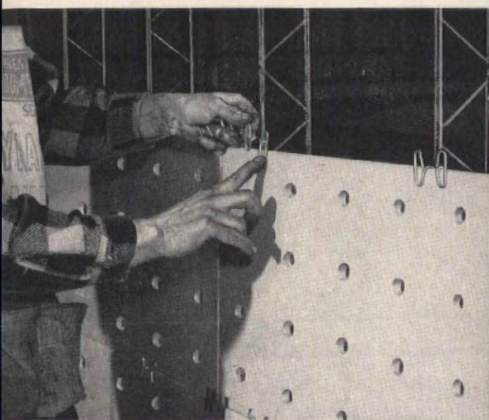
TR-1 clip attaches easily, holds perforated ROCKLATH plaster base firmly in position.
