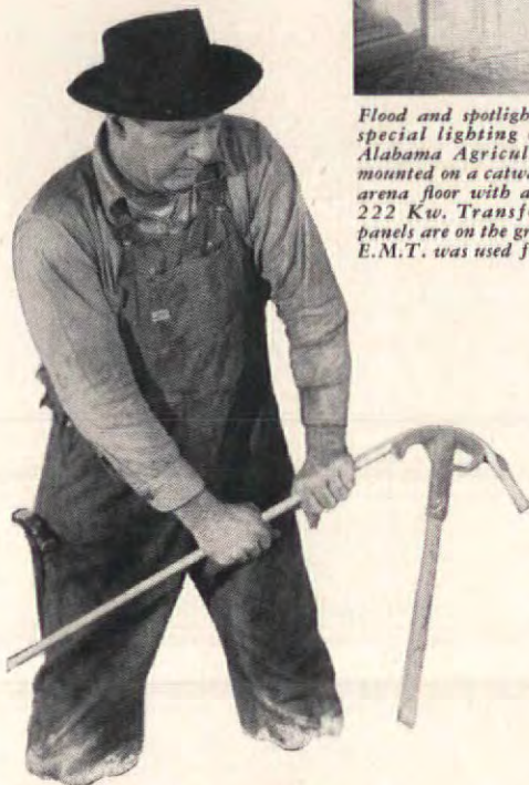
Smooth bends are made accurately and quickly, using the Republic one-piece calibrated bender, with "Inch-Marked" E.M.T.
