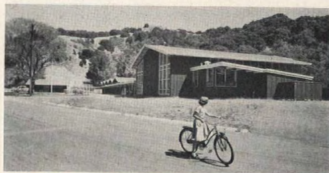
Manor Elementary School, Fairfax, Cal.; John Lyon Reid, architect. Gabled roof provided fresh approach to bilateral lighting, gave each class a "house" of its own in structure designed for strict economy
