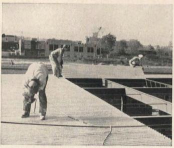
1. STEEL SHEETS ARE QUICKLY PLACED AND SECURED by welding or by clips attached to top of joist as soon as joists and beams are erected. Positive attachment of tough-temper sheets gives added rigidity to roof framework, provides immediate working platform. Tufcor and Corruform are galvanized for permanence, give better service than ordinary painted metal deck.
