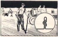
A special Robertson clamping tool mechanically fastens the side laps together, forming a steel fire barrier that remains intact as long as the structural supports are in place.
