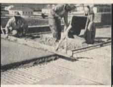
2. INSULATING CONCRETE FILL IS PLACED on the deck after it has been welded to the beams and a light mesh has been rolled into position. A tight solid base is provided by Tufcor and Corruform, retaining cement paste in the slab and insuring maximum strength. Granco Vent Clips (attached to side lip of the sheet) prevent vapor pressure build-up.
