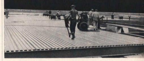
The many unique features of Robertson Q-Deck make it of special interest to the architect and engineer who is concerned about the fire hazard aspect of his flat roof design. To begin with, Robertson Q-Deck is designed with tight side and end laps to eliminate the need for an inflammable vapor seal. Its two-foot width and long span characteristics mean fewer joints, and its zinc-coated surface (or basic Galbestos) eliminates the need for field painting.
