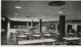
Venturi-Flo Diffusers in the ceiling, Uni-Flo Return Grilles in the sidewalls provide fresh, conditioned air in the cafeteria.
