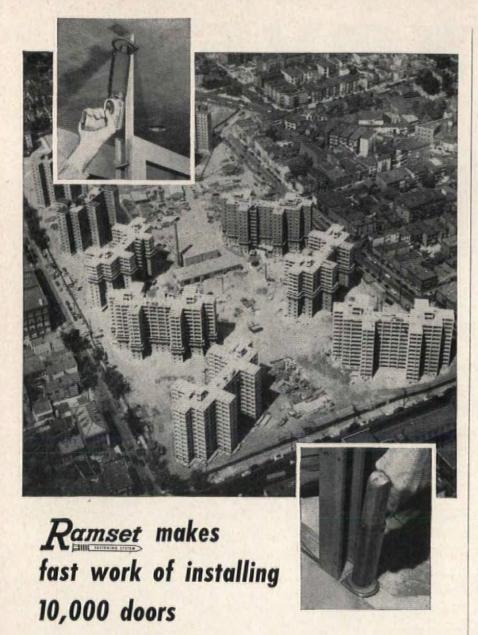
Speed and economy resulted from the use of RAMSET SYSTEM to anchor 10,000 interior doors top and bottom in the low-rent housing project at Newark, N. J.
