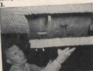
FIBERGLAS insulation, Type PF-613, 2" thick—bonded to concrete ceiling using MIRACLE PRONGED ANCHORS at Radio City Studio 6B, New York, N. Y. CONTRACTOR, William J. Scully, Inc., New York, N. Y.
