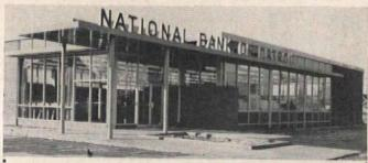
National Bank of Detroit. Architects: Hawley, Ellington & Day, Detroit, Mich. Featured is Alumiline Curtain Wall Construction (60% of total wall area). The Curtain Wall contains both glass and porcelain insulating panels, with the construction based on 2" x 5" tubing. This Alumiline Curtain Wall was sent to the job completely prefabricated.
