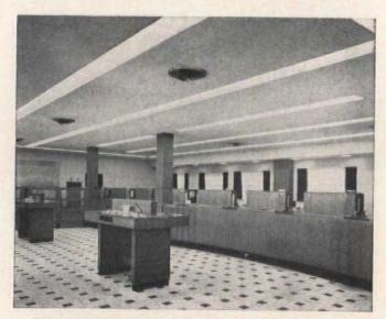
Typical Interior of a modern bank. Note location of diffusers in rows along acoustically treated ceiling to give good distribution of air to all areas.
