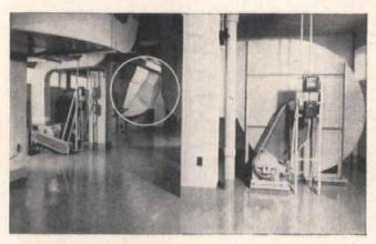
These large fans are floated on rubber vibration pads, and one fan(left background) has canvas sleeve to absorb vibration noise before it can enter ductwork.
