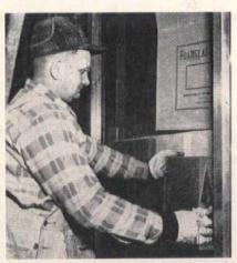
Workman easily cuts FOAMGLAS blocks to fit between steel frame members of sub-structure.
