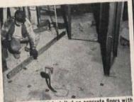
WOOD RUNNERS installed on concrete floors with MIRACLE ADHESIVE and MIRACLE ANCHOR NAILS to support 2" solid partitions. Washington Circle Apartments, Washington, D.C. GENERAL CONTRACTOR, Charles H. Tompkins Company.
