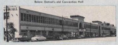
Construction above and below vision strip on Woodward Avenue side of building consists of enameled glass outer face, air space vented for condensation drainage, FOAMGLAS adhered to transit and backed up with composition wall board. End wall construction is similar except that enameled porcelain is used in place of enameled glass for the outer face.
