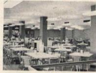
CAFETERIA. 4 Lamp 40 Watt "Skylouver" fixtures with 45° x 35° shielding. Pendant and flush mounted on 10\\\\^2\end{c}' centers to provide average of 35 maintained foot candles. Electro Silv-A-King No. 1045 with styrene louvers and side panels.
