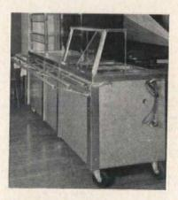
55. The Silvercraft Inc. portable cafeteria counter, made up of three of the company's standard units bolted together and riding on swivel rubber-tired casters, includes hot and regrigerated units said to reach desired operating temperatures from 3 to 5 min. after the switches are turned on. (Louisville, Ky.)
