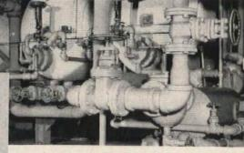
Among nearly 3000 Jenkins Valves, controlling all lines, are these Iron Body Gate Valves on steam condensate lines of hot water system.
