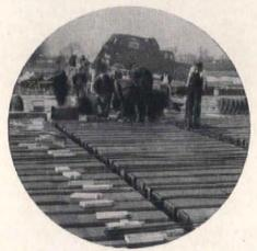
One-way Ceco-Meyer Steelforms also save steel and concrete, thus reducing dead load.
