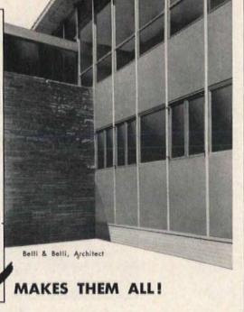
The burden of designing for porcelain enamel walls is no longer yours! ERIE has developed a range of panel designs adapted to curtain wall, window wall and spandrel treatments using any of a variety of structural supports. You can use filled panels, laminated or insulated panels—as designed or modified to your requirements.
