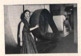
**Basement** — Sirocco Fans circulate fresh, dehumidified air. Total rating of American Blower equipment in building is 770,378 cfm. Gross floor area is 503,000 sq. ft.
