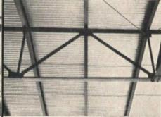
4. RESULT: A FIRE-SAFE ROOF WITH AN ATTRACTIVE UNDERSIDE. Clean, smooth Tufcor and Corruform steel sheets may be left exposed underneath, using the bright galvanized surface for light reflection, or if desired, any normal ceiling treatment may be applied including paint, suspended plaster, sprayed-on acoustic plaster, etc.
