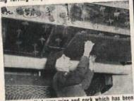
Plaster applied over wire and cork which has been attached to aluminum ducts using MIRACLE AD-HESIVE and MIRACLE SPINDLE ANCHORS at John Hancock Mutual Life Insurance Co. Building, Boston, Mass. ARCHITECT, Cram and Ferguson. BUILDER, Turner Construction Co.
