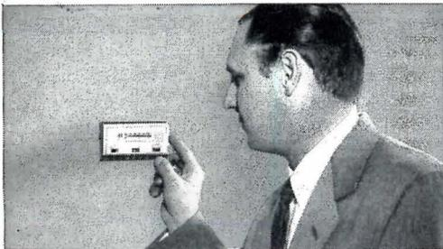
**ONE-POINT THERMOSTATIC CONTROL.** Home-owners can change from summer cooling to winter heating by flicking a switch and setting temperature wanted. No fiddling with dampers.
