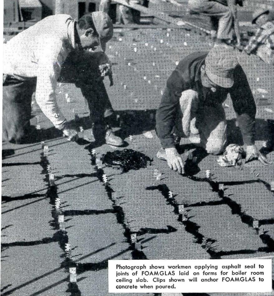
Photograph shows workmen applying asphalt seal to joints of FOAMGLAS laid on forms for boiler room ceiling slab. Clips shown will anchor FOAMGLAS to concrete when poured.
