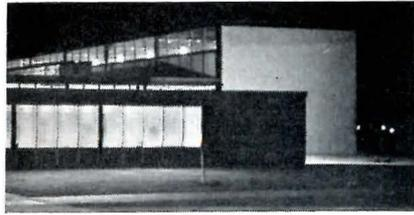
*Walls are masonry between steel columns whose flanges are exposed inside and out; this device breaks the masonry into panels small enough to prevent expansion cracks, eliminates expansion joints*
