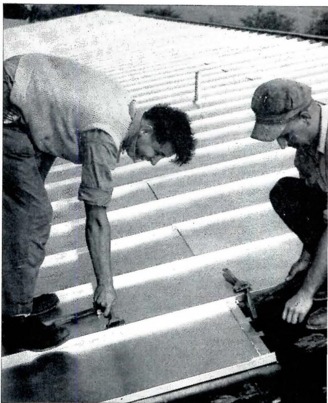
**INSTALLING** the standing-seam USS Stainless Steel roof on the new Walnut Grove School. The roof was laid on double-coated asbestos felt with each cross seam carefully caulked before the upper sheet was installed.
