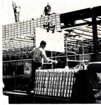
*Pre-cast brick panels are stacked on truck and delivered to the job site*
