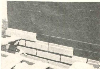
*Nailon Brick* is the facing on the house shown at right above. The 1-in.-thick "bricks" are of real clay composition and are the same as actual bricks in appearance, texture, size and mortared joints. They can be *nailed directly* to any nailable surface: plywood, wood siding, asbestos siding, stucco and concrete block.
