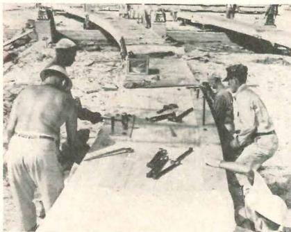
The arches vary in depth from 26 in. at the base to 46 in. at the point of maximum stress to 22 in. at the crown, where the height is 80 ft. Each arch weighs over 15 tons, contains 17,000 board ft of Southern pine lumber and measures 340 ft along its circumference. Wood decking, 3½ in. thick, attached directly to the arches eliminated the need for purlins and other bracing. Architects of the Fronton were Spicer and Gehlert of Daytona Beach. Structural engineer was J. G. Moore.
