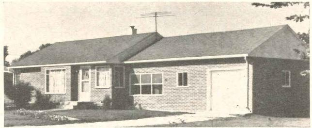
Lightweight, cellular concrete supports house at left; thin brick units are nailed onto house at right
