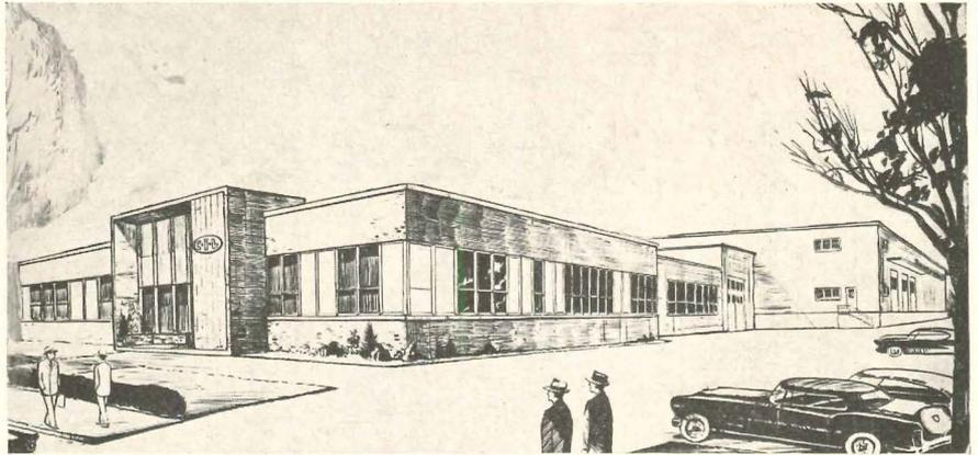
A distributing center is planned for Halifax by Canadian Industries (1954) Limited; the building, which will have a steel frame "sheathed" with tile, will contain offices and warehouse space. J. Philip Dumaresq, of Halifax, is the architect
