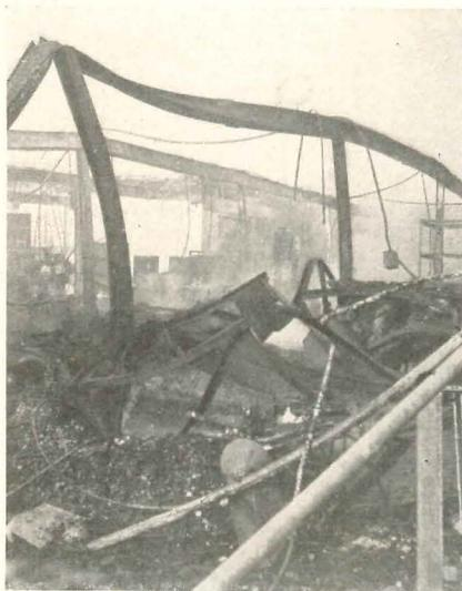
McKay-Davis Chemical Co., near Toledo, Ohio. Burned Sept. 14, 1955. Loss: \$309,000. Contributing causes: No sprinklers or automatic fire detection system, unprotected horizontal openings, fire doors blocked open, flammable liquids.
