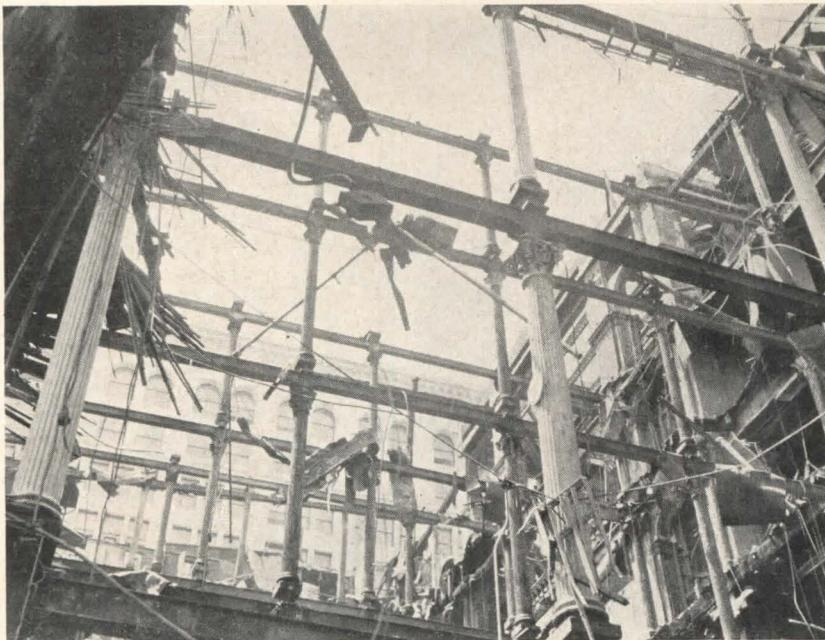
*While fire has destroyed the wood joists, cast iron columns and wrought iron beams stand straight and true*
