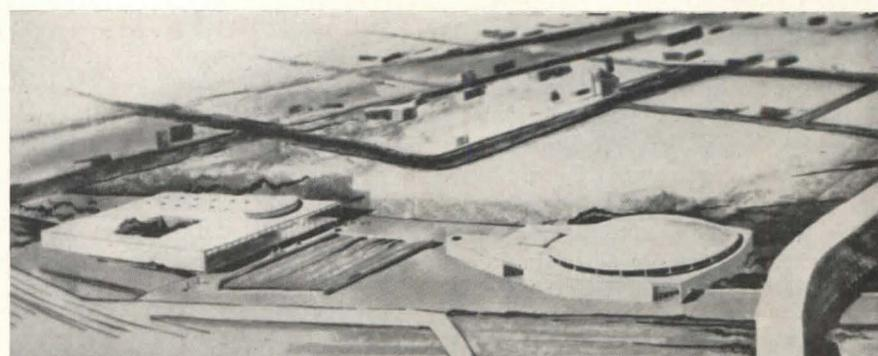
The hill was shaped as shown above, covered with plywood and reinforcing steel and then scooped out from under the shell after the concrete had set. Auditorium will be part of cultural center at right
