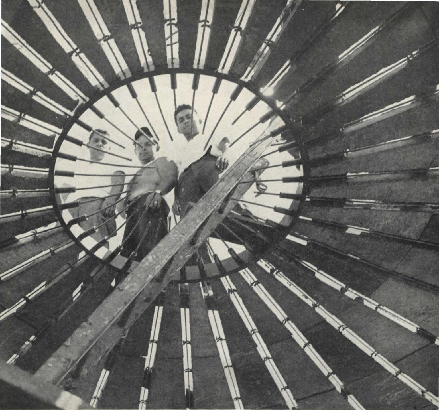
*can be seen from view under roof. Notice the steel cables projecting through inner steel ring, held by wedge fillings*
