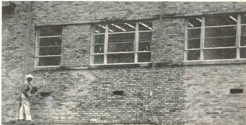
*Silicones are applied on large areas by means of a low pressure spray in a flooding action so as to insure thorough treatment*
