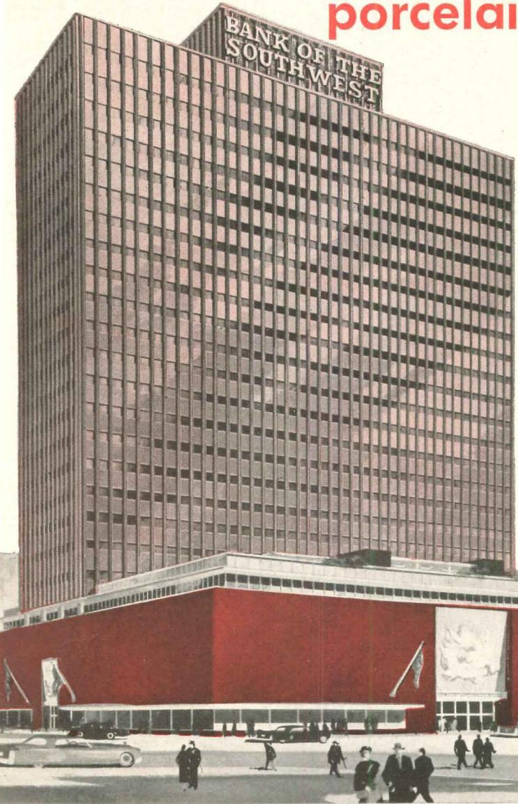
Recently completed, the Bank of the Southwest stands as the tallest welded structure in Houston, Texas. One of the many interesting features of this building is the extensive use made of lightweight materials in the superstructure—especially in the vertical trim on the mullion panels. Here, 32,892 linear feet of aluminum, finished with Du Pont porcelain enamel, were used with color selection to harmonize with the red granite base.
