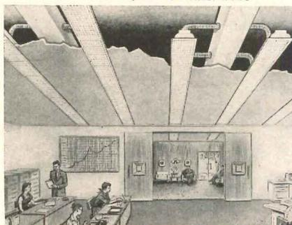
LIGHTING AND AIR CONDITIONING are now possible from the same fixture with the *Multi-Vent Trofferlite*, a combination light fixture and air diffuser which is adaptable to any drop-type ceiling. The fixture uses an air pressure displacement principle instead of high-velocity injection, so temperatures are said to be easily balanced and to stay uniform throughout the area. As shown in the drawing, flexible tubing feeds from the main ducts into the tops of the light
