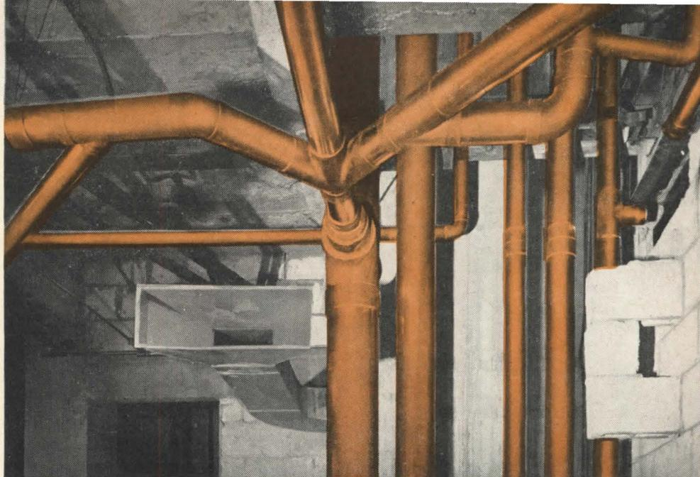
**Tube and fittings fit in standard partitions.** A 3" copper tube stack with fittings can be installed within a standard 4"-wide stud partition.
