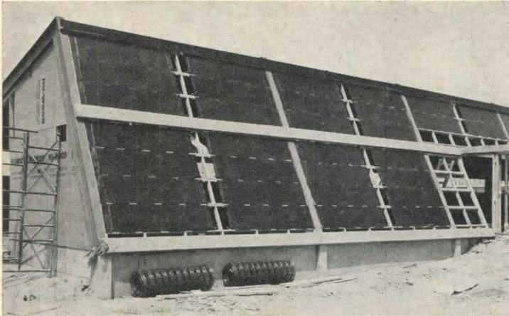
Black aluminum collector panels enclose integral water channels  $\frac{1}{2}$  in. wide by  $\frac{1}{8}$  in. deep
