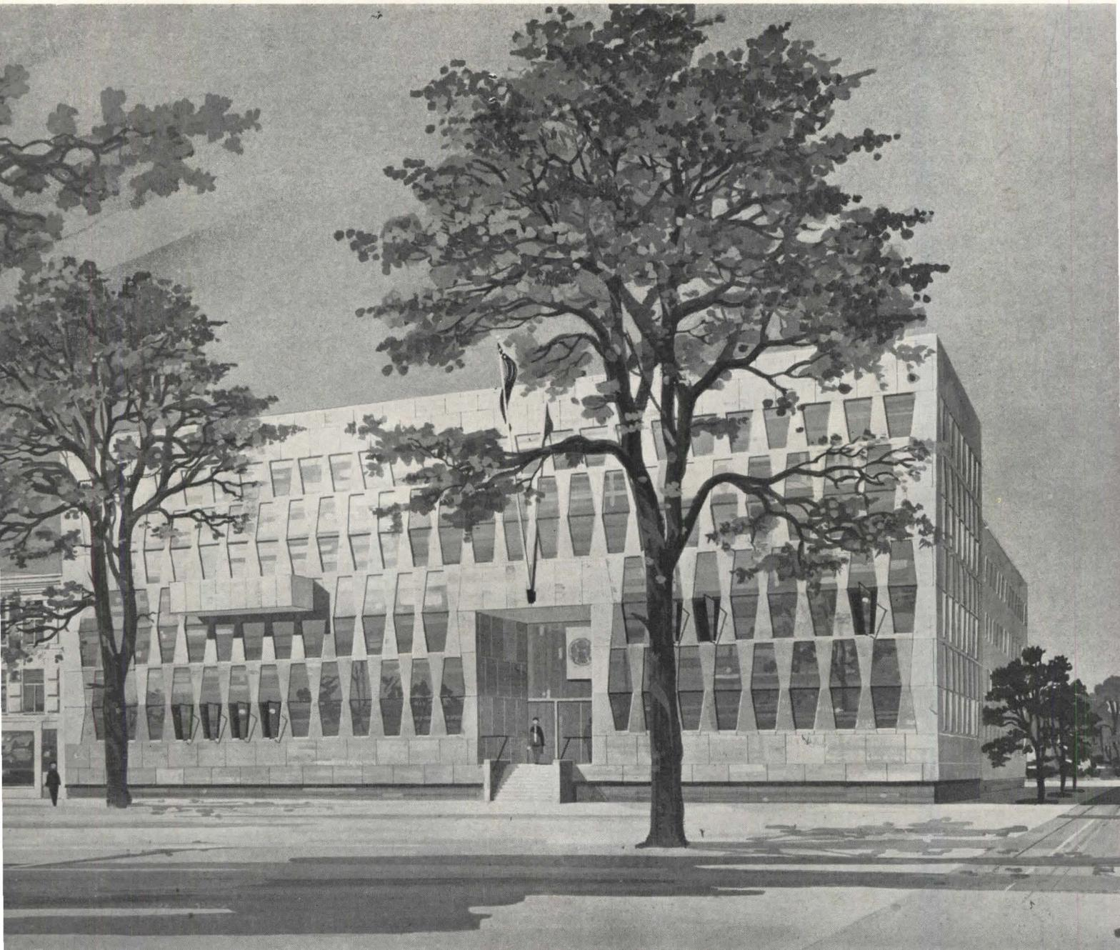
the sides of the openings were chamfered to ease the flow of diagonal stresses. The result is an over-all fenestration pattern in a wall that looks and acts like a unit. Also, there is now the opportunity to group the openings into plastic forms, as was done in the elevation at bottom right.
