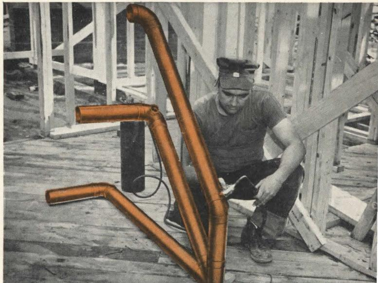
**Lightweight for easy, fast handling.** This preassembled section comprising about 13 feet of copper tube and 5 solder-joint fittings weighs only 35 pounds, is easily handled by one man.
