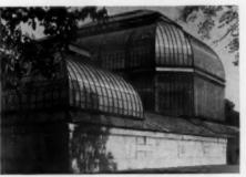
Despite the warm, moist air in the gardens, the all-aluminum superstructure is in excellent condition. Here is one of the earliest structural applications of aluminum. No effort has been made to maintain the surface appearance, yet even in an atmosphere trying to most metals, no corrosion problem has been experienced.
