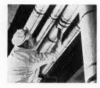
The makers of Hellmann's Mayonnaise first used Styrofoam\* (a Dow plastic foam) in 1952. That was to insulate egg-storage rooms. The results have been so satisfactory that when Best Foods planned a new unit for making salad oil, Styrofoam was specified for  $40^{\circ}$  insulation in the winterizing cells (see illustration).
