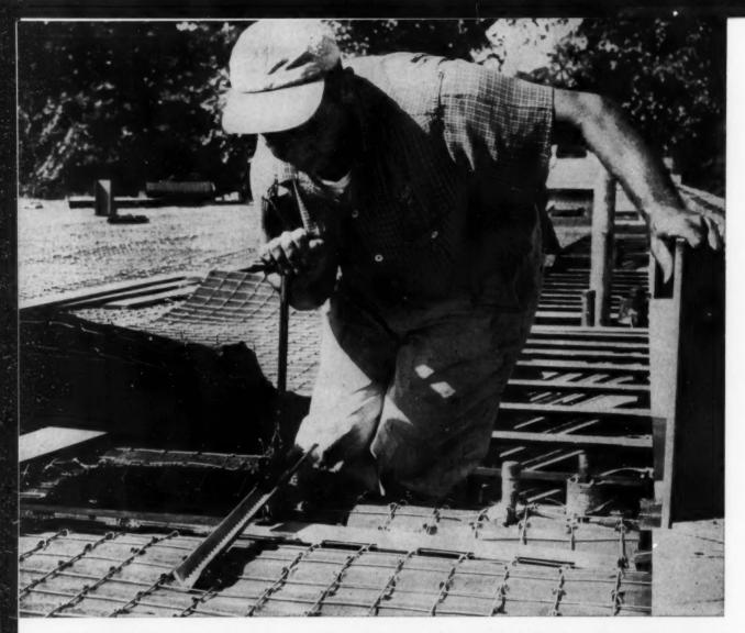
A better roof or floor slab results at lower cost when architects and contractors agree on Steeltex Floor Lath, the wire mesh reinforcing that carries its own water-proofed form right on its back. Steeltex can be unrolled, stretched as in the photo above, and clipped with simple tools by workmen without previous training.
