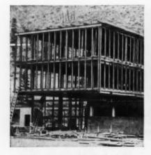
Ready for the Lupton Windows. Completed installation of outer mullions before erection of Lupton Windows. Notice outstanding simplicity the windows themselves become the walls in this all-Lupton installation.
