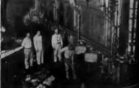
OLD SOILER was a coal-fired HRT model — typical of many replaced by modern Cleaver-Brooks oil, gas or combination oil/gas fired boilers.
