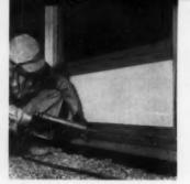
Sealing Around Mullion and Sill Joint in an aluminum-porcelain window wall
