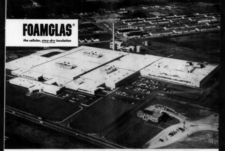
The moisture-proof structure of FOAMGLAS proved important in exterior corewalls of Lorillard's Greensboro plant. It permitted use of a ¼-inch space for condensation accumulation between insulation and exterior brick. Only FOAMGLAS can guarantee no loss of insulating value from moisture drainage across its surface. Architects-Engineers: Lockwood Greene Engineers, Inc., New York.
