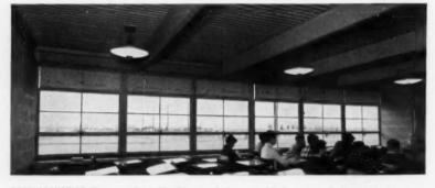
GOOD ACOUSTICS. Tests conducted by Riverbank Acoustical Laboratories indicate that Structur-Acoustic system with 21/2" slab provides Noise Reduction Coefficient of .80. Clean, corrugated underside of Structur-Acoustic reflects light, can be painted to matching color scheme. Hard surface won't dent, stays attractive. Heat loss is kept to minimum with U factor in excess of 0.14. Firesafe system protects both building and contents, helps reduce owner insurance costs.
