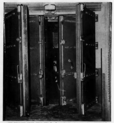
JAMISON sound reduction doors lead in engine test cell
