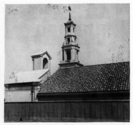
Monel protection. Tower sheathing, flashings, parapets, bulkheads, drainage system and skylight frames of Regina Pacis Votive Church and adjoining parochial school are all fabricated of .021" Monel Economy Roofing Sheet. Corrosion resisting and long lasting, Monel weathers uniformly where exposed. Architect: Anthony J. DePace, 151 W. 46th St., New York 36, N. Y. Sheet metal contractor: John Schneider Roofing Contractors, Inc., 1056 Cypress Ave., Brooklyn 27, N.Y.
