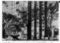
This Stainless-covered apartment building will never lose its luster. More than 60% of its exterior surface is made up of spandrels fabricated from Republic ENDURO® Stainless Steel. That means it will stay vivid and attractive for life. High resistance to rust and corrosion reduces maintenance costs. And there's a saving in weight. Send coupon for ideas on how ENDURO Stainless Steel can help you. Interested in windows, joists, stainless spandrels? See Republic.
