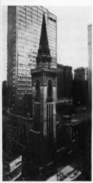
This 80-foot-high spire, rising 259 feet above the street, is darkened from 31 years of weather exposure. The aluminum is as sound as the day it was installed. Note 30-story Alcoa Building with its aluminum curtain wall in background.
