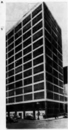
This building is considered to be the first true application of aluminum in curtain wall construction. There's no masonry surface at all above the first floor. All of the glass and metal panels are held in aluminum frames.
