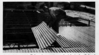
EASY TO PLACE. Tufcor sheets arrive at the job site bundled and cut to fit framing. No measuring or cutting is needed! After sheets are plug-welded in place, they provide a strong structural deck and a convenient work platform for trades. In the finished roof system, Tufcor acts as a vapor barrier, keeps insulating concrete dry so it maintains its insulating properties, saves on costly fuel bills.
