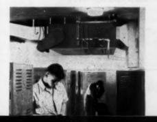
FOR HIGH-CHILINGED SPACES, TRANE Unit Heatern with exclusive louver cone diffusers are often the answer. Two-thermostat control traps otherwise wasted heat near ceiling, blows it down to save fuel.
