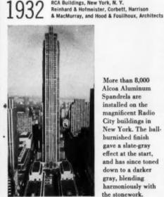
More than 8,000 Alcoa Aluminum Spandrels are installed on the magnificent Radio City buildings in New York. The ballburnished finish gave a slate-gray effect at the start, and has since toned down to a darker gray, blending harmoniously with the stonework.
