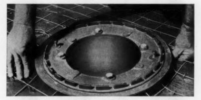
You eliminate messy drip-through on the floor below when you use Steeltex. Mesh and water-proofed paper backing can be fitted right to the edges of objects like this sump on the roof deck.
