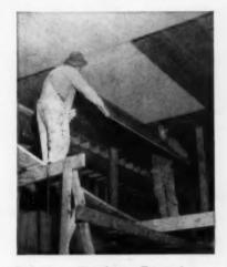
Stripping ceiling forms. Exposed concrete surfaces, both inside and out formed against 5%" fir plywood, were painted direct after minimum of rubbing, eliminating plastering.
