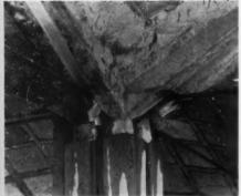
Shell being guided into position alop columns. Note temporary tie rod above, permanent tie rod below (with turnbuckle). Tie rods across interior shells are required because of the possibility of unbalanced load conditions; otherwise thrusts from shells would cancel
