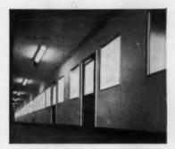
Johns-Manville flush or glazed partitions are furnished and erected by J-M's own Construction Department, complete with doors, door hardware, glass and trim.
