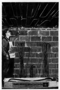
Approximately 3200 Anaconda Panel Grids were installed in ceilings throughout the Kenmawr Apartments. The PG's came to the job in handy cartons shown, ready to open out and fasten to the metal lath by tie wires.
