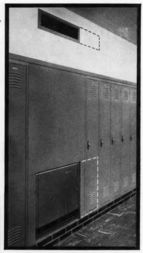
Here's how the use of Type W coils with hot water can reduce unit size. Dotted lines indicate space steamcoil units of equal capacity would need.
