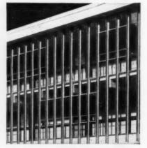
Adjustable ventilation. Projected in at bottom or out at top, these Lupton Windows provide immediate controlled ventilation with maximum light, are tight-fitting and rattle-free.
