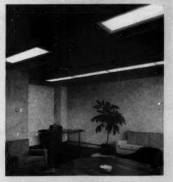
There are 391 fixtures, using 1,564 square feet of LUCITE, illuminating about 30% of the total floor space in the building. The LUCITE is installed in a single frame of steel hinged to the fixture. The Housing Center has an average of 45 foot-candles, as opposed to the 30 foot-candles issually found in office buildings.
