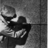
Sealing Horizontal and Vertical **Expansion Joints between cast** stone and panels.
