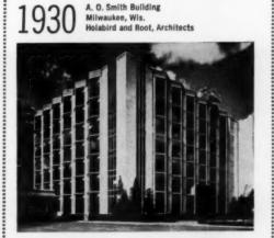
Still modern looking and attractive after more than twenty-five years, this structure makes fine use of large aluminum window frames and pilasters. The interior applications of aluminum in main lobby are outstanding.
