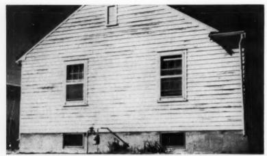
Blistering and peeling paint is one of the most common types of damage caused by the collection of excessive vaner in the side walls.
