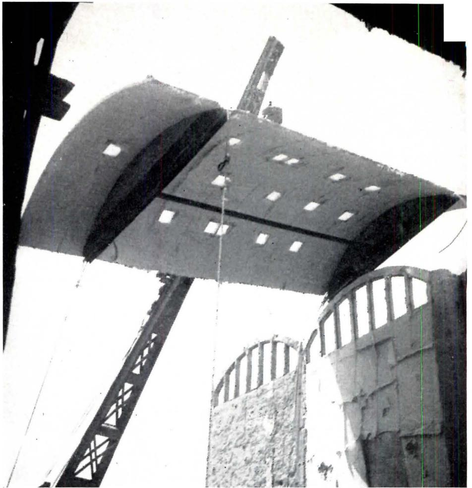
*Openings for doors and windows — and even glazed skylights as in the shell at right — are formed into the elements as they are cast. To eliminate tie rods and speed erection, column capitals and upper wall sections follow the curvature of the shells they support.*
