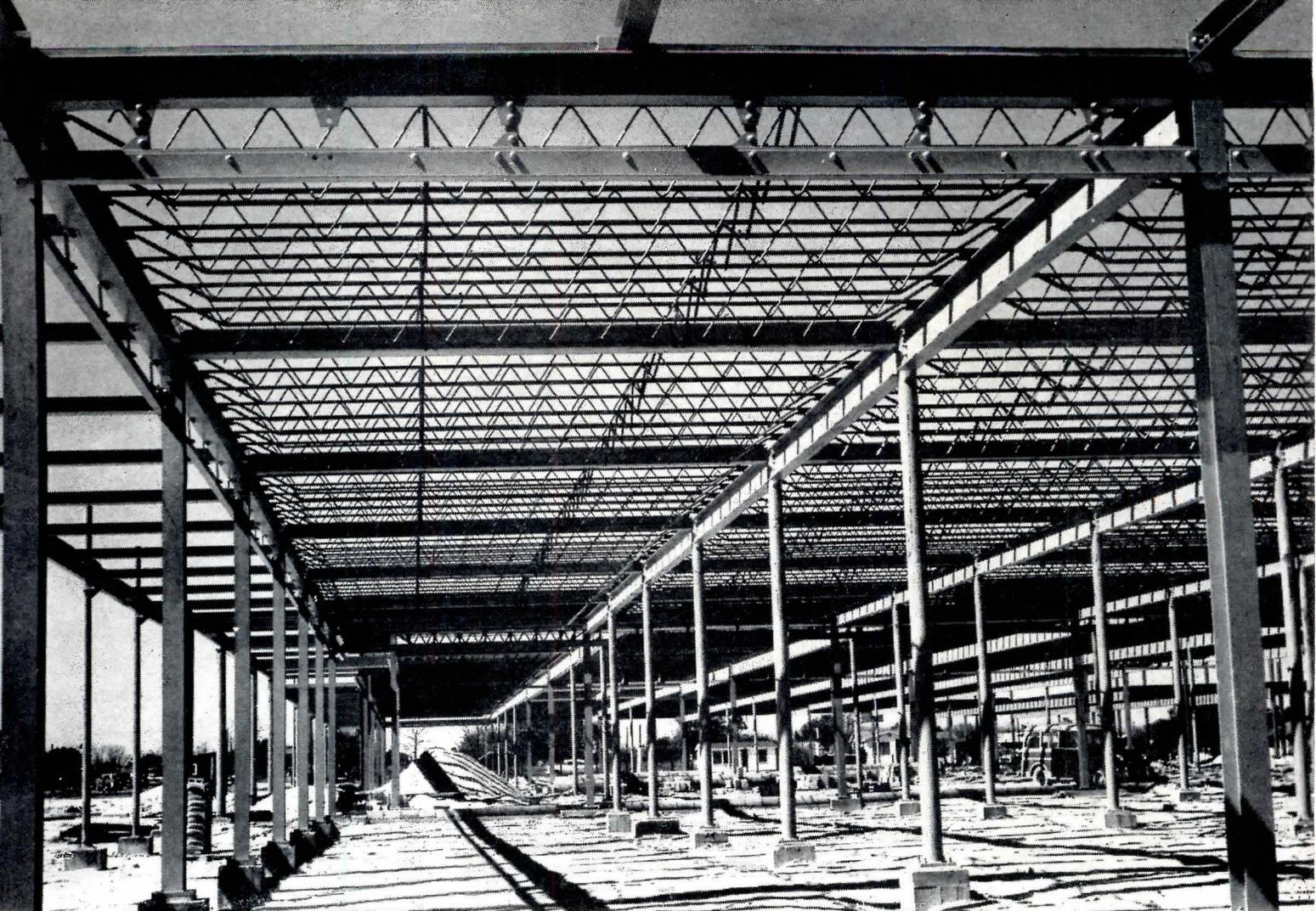
THE TOWN AND COUNTRY PLAZA SHOPPING CENTER, Pensacola, Fla., used 1,825 tons of structural steel, including 448 tons of AmBridge Steel Joists—all fabricated and erected by American Bridge.
