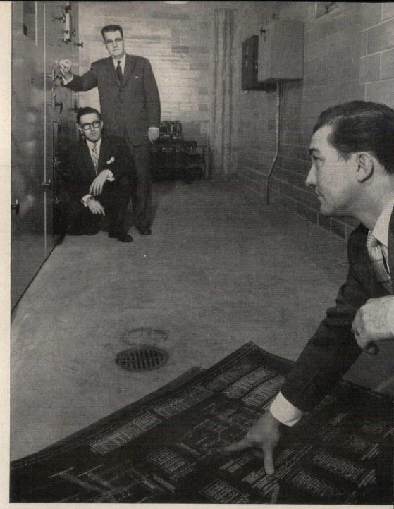
Contractor and engineers discuss metal-clad switchgear employing preferred-emergency incoming line transfer arrangement.
