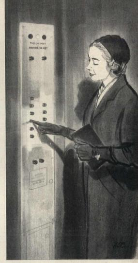
IN 1958-The Travelers will have an entirely automatic elevator system, without attendants. The passengers themselves will press their floor buttons in the car and the doors will operate automatically without human supervision. Service rendered will be more efficient, fasterand even safer.
