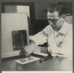
4 Second analytical weighing to determine corrosion weight loss
