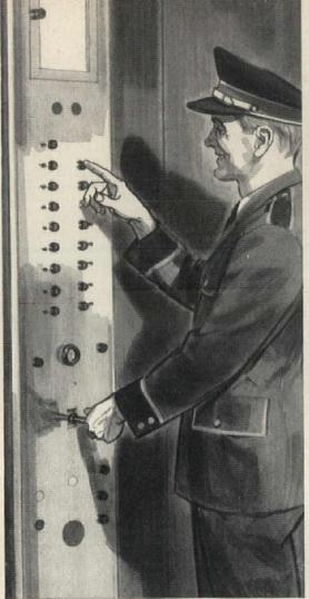
IN 1946-modernized Westinghouse Elevators were automatically operated from pushbuttons in the car. Attendants were still required, however, to press the floor buttons and to initiate the closing of the power operated elevator doors.
