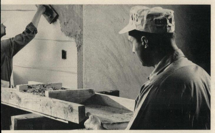
Easy to install. Handsaws and other common tools readily cut a board of Styrofoam sharp and clean. Or, Styrofoam can be scored with a jackknife and snapped off to any desired size. Easy to apply to any masonry surface with Portland cement mortar or other recommended adhesives.
