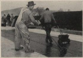
Lexsuco's semi-mechanical method is fast for medium or small jobs. Ribbons of adhesive are applied with spreader and rolled into a solid coat for securing Koroseal. Then insulation is embedded into the ribbons of adhesive spread over the Koroseal. It's like a production line! A manual method also is practical for small jobs using pouring can instead of spreader.
