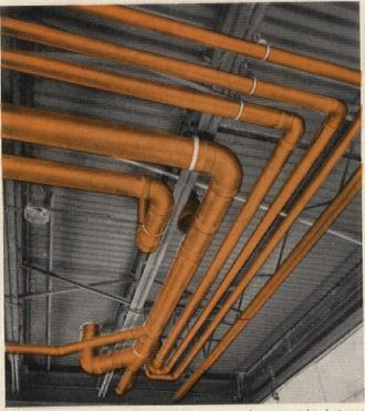
WATER PIPING and sanitary drainage lines of copper tube between floor and ceiling. The light weight of copper tube makes overhead work like this easier and faster. Copper tube with cast-brass solder-joint fittings was used throughout the 5-story building for the sanitary drainage system.
