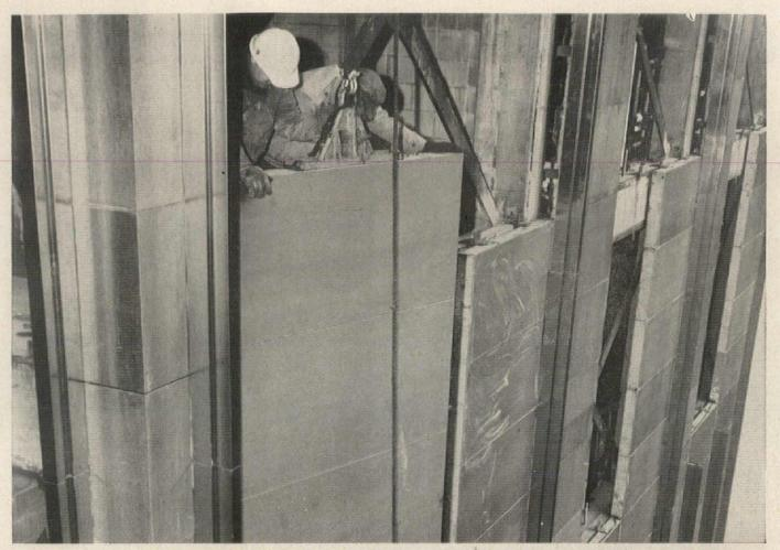
Panels are hoisted into position from street level and secured to the steel skeleton. The 13' x 5' panels are faced with stainless steel and contain Styrofoam, the insulation with lifetime insulating efficiency. Architects-Engineers: Skidmore, Owings & Merrill.
