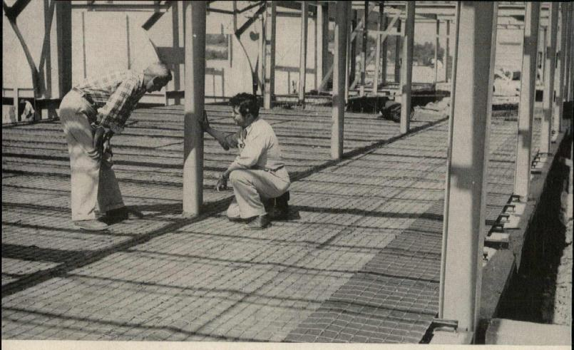
Fastest coverage with Steeltex. Steeltex roll, 125 feet long and 4 feet wide, unrolls quickly and is easily cut to fit around irregular-shaped objects like the steel
