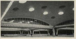
Factory in Brynmawr, England has two sets of ceiling openings, with same geometry, one for daylight, the other for electric light. Good example of thoughtful lighting for a thin shell
