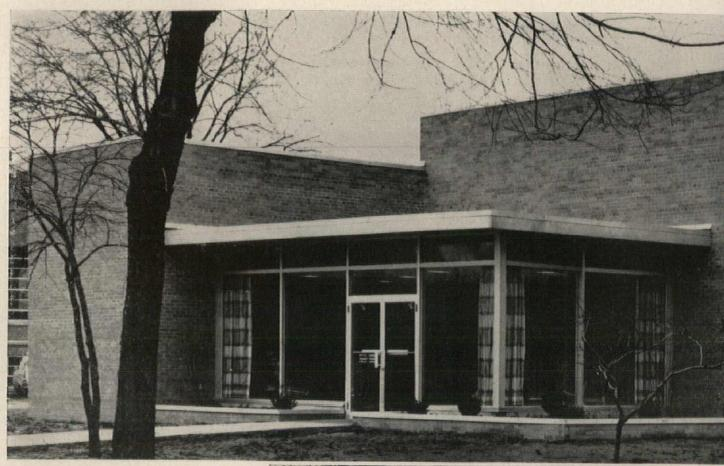
Photo from exterior. Warren City Schools Administration Building, Warren, Ohio, is two stories high with the first floor line five feet below grade and second floor line five feet above grade. Entrances are located midway between floors.
