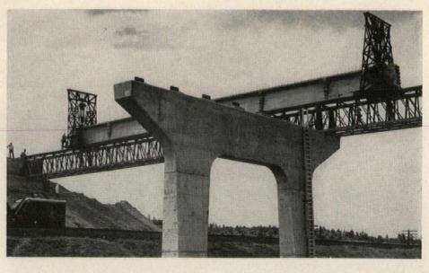
straight forward into their final position on the piers. The unique handling method developed by the contractor involved the use of two gantries which rolled on rails along each side of the casting beds. These rails extended to the edge of the bridge abutment and on across the tops of light triangular steel trusses over the first and second spans, forming a temporary "bridge" from which the girders could be placed.
