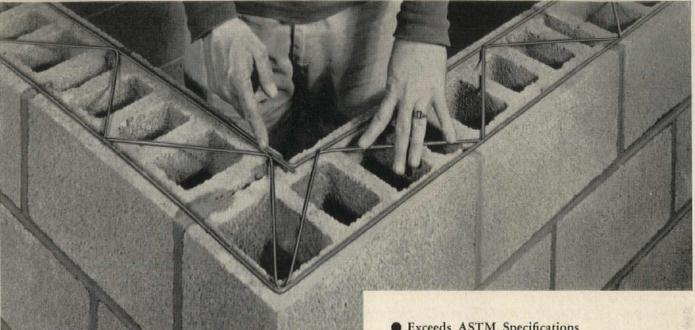
Dur-O-wal is custom-fabricated to lay flat and tight in the mortar bed. Research tests demonstrate that "a wall with five courses of reinforcing is 260% stronger than non-reinforced masonry walls with Class B mortar and 245% stronger than walls constructed with Class A mortar." "Where strong mortars are used, the strength of the wall increases as the amount of steel increases." Dur-Owal, reinforcing pioneer and recognized standard of quality, is preferred for its unexcelled performance.
