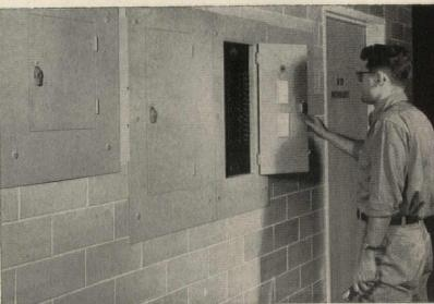
Westinghouse Type NLAB Quicklag® breaker lighting panelboards. A total of 42 lighting panelboards and 10 power distribution panelboards are installed in the hospital.
