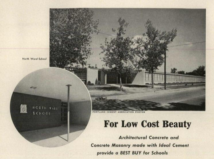
An economical dual application of concrete was developed for the construction of the North Ward Elementary School in Superior, Nebraska. On both the inside and outside of this handsome school building, concrete walls were left exposed.
