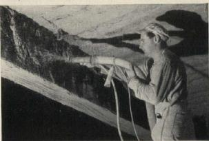
Zonolite and modern plaster machines were used to fireproof steel floors and beams. Plastering Contractor: E. B. Carley & Company, Jackson Heights, New York.
