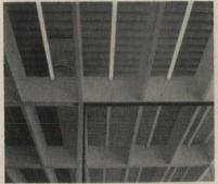
Louvered grid in Connecticut General Bldg. by Skidmore Owings and Merrill hides fluorescent tubes, ducts and diffusers; provides sound control
