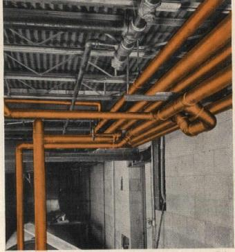
PARTIAL VIEW of compact copper tube installation in basement. Tight working space presents no problem with copper tube and solder-joint fittings. Architect: John N. Marx, Chicago. General Contractor: Cornelius Pitt and Company, Chicago and South Bend. Mechanical Contractor: Allied Plumbing & Heating Co., South Bend.
