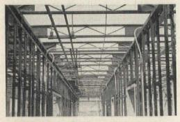
In addition to V-BEAMS, MACOMBER "nailable" LOAD-BEARING PARTITIONS were supplied for use in corridors of offices, classrooms and dormitories.
