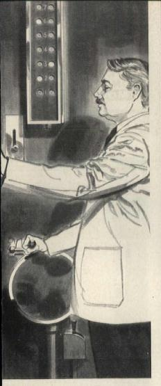
1922—elevators in The Travelers home ice were manually operated by means of a switch inside the elevator. The elevator ors were opened and closed manually. The curacy of leveling at the floors depended upon skill of the attendant.
