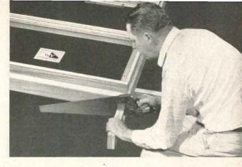
Simple, error-proof construction! Just cut two load-bearing struts to fit header construction. Nail Strutwall to adjacent studs, tilt up with the wall. This cuts installation steps twothirds. Practically eliminates chance of carpentry errors and callbacks.
