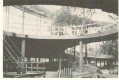
The roof of the U. S. Pavilion utilizes a bicycle-hub principle to achieve a clear span of 350 ft, making it the largest circular building in the world without interior columns. The hub is open to the sky above a central pool 133 ft in diameter; exhibition space surrounds the pool on two levels. Eleven willow trees found on the site have been preserved within the pavilion.
