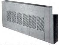
Inductor Units for cooling or heating multi-room buildings. Can be connected in series. Mounted vertically or horizontally (without excessive casing depth). Wide range of sizes.
