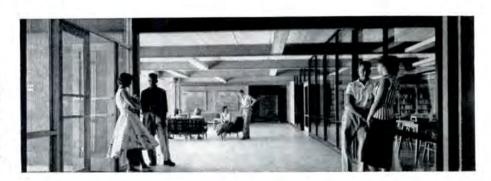
STUDENT COMMONS and lobby area at the recently completed Baldwin High School in Baldwin, N.Y., features a random arrangement of incandescent globes suspended at varying heights to add a decorative accent in the center of the large open area. Overall illumination is provided by can-type downlights mounted in regular rows on a dark-painted ceiling
