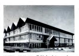
DENVER, COLORADO: Folded plate roof on Denver-Chicago Trucking Company's new office building is of thin-shell concrete. Toll and Milan, architects; Ketchum and Konkel, structural engineers
