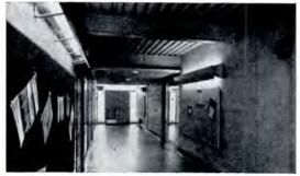
At Northport, a dropped ceiling at the end of the hall conceals mechanical equipment, and heightens the contrast between the uneven light from wood-baffled fluorescents over display boards in the corridor itself and the brightly-lit entrance at the end
