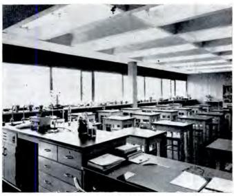
MULTIPLE USE OF STRUCTURAL MATERIAL AND FORM: in the Conard High School, West Hartford, Connecticut, reinforced concrete pan construction enabled exposed structural ceilings throughout for structural, finish, acoustic, and esthetic purposes, and provided built-in light baffles to house inexpensive fixtures. Nichols and Butterfield, Architects
