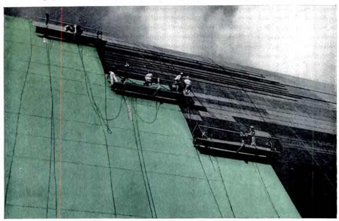
Engineering study at Lakehurst recommended industrial corrugated aluminum roofing for three reasons: it is comparatively inexpensive and provides a durable and permanent-type roofing; it requires lowest expenditure for maintenance; it can usually be installed without changes in the existing structural framework.
