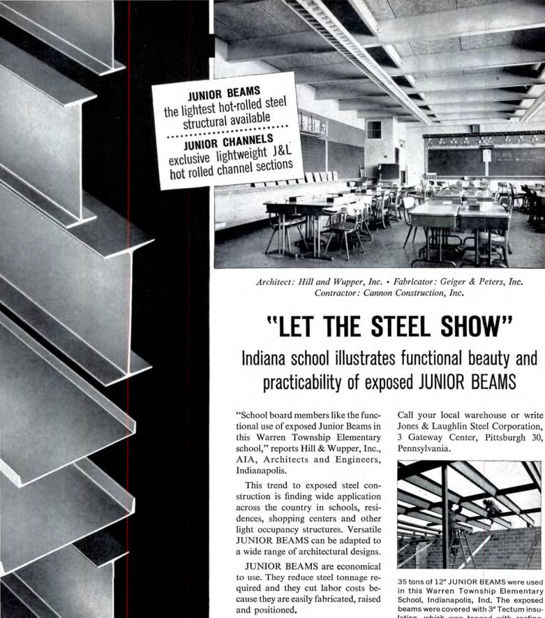
in this Warren Township Elementary School, Indianapolis, Ind. The exposed beams were covered with 3" Tectum insulation, which was topped with roofing. Modular design has windows and columns on 4' centers.
