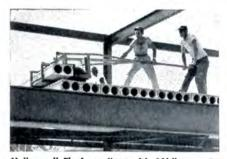
Hollow-cell Flexicore floor with 1½" concrete topping has 3-hour fire rating from national authorities. Needs no fireproofing on ceiling.
