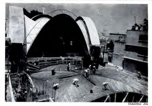
Church San Antonio de las Huertas, Enrique de la Mora, Architect, is roofed with three groined vaults. Over the crypt are two star-type vaults of a more complicated nature, formed by combinations of hyperbolic paraboloid sections
