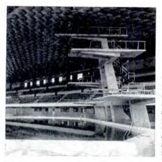
The Tokyo Metropolitan Indoor Swimming Pool, Masachika Murata and Associates, architects, is of reinforced concrete, with sprayed-concrete-coated steel roof trusses spanning 162½ feet. The building was completed this spring for the Third Asian Olympic Games. At left, 20- by 25-meter diving pool, 20- by 50-meter swimming pool, and grandstand seating 4000 people. Below, main entrance and offices.
