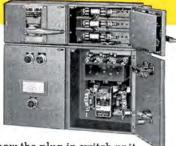
Notice how the plug-in switch unit is mounted directly above the starter, permitting interlocking. The starter cannot be opened when the switch is in the "ON" position.
