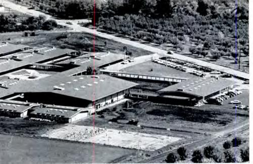
MODULAR COORDINATION: Miramonte High School in California (left), is the first consructed example of the use of Ernest J. Kump's Basic Space Module. This is based on the economic advantage of repetitive components: whole buildings of identical structural, mechanical, and electrical design are repeated many times in a large school
