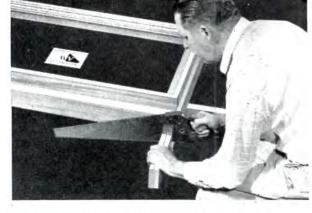
Simple, error-proof construction! Just cut two load-bearing struts to fit header construction. Nail Strutwall to adjacent studs, tilt up with the wall. This cuts installation steps twothirds. Practically eliminates chance of carpentry errors and callbacks.
