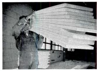
"SEVERAL 8-FOOT BOARDS of lightweight Styrofoam can be easily carried to the job site by one man. In just one stroke, Styrofoam is cut to 48-inch lengths using the sharp edge of
