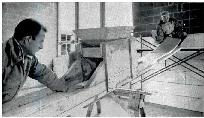
"AN AUTOMATIC MORTARING JIG evenly coats each 4-foot section of Styrofoam with %" of mortar. The boards are pushed manually through the box and passed on to the installation man who puts them into position. Styrofoam adheres directly to the masonry, eliminating furring. This operation is so fast and simple that we achieve time reduction and cost savings by its use."
