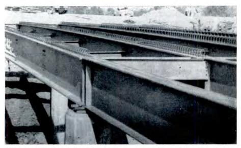
SPIRAL SHEAR CONNECTORS. Tie of steel beam to concrete slab is also performed with a round bar, wound into a helix which is welded to the beam at spots where it touches
