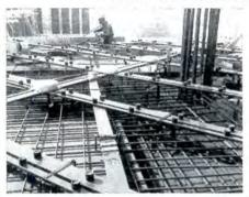
Underfloor Electric Distribution System Features Diagonal Layout
