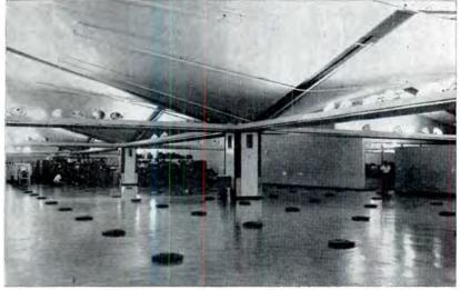
1500 access holes at 10-1/2 ft centers in the manufacturing floor slab make available any service at any point. Services include natural gas, some rare gases, water, electricity, communications and comfort conditioned air
