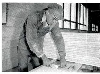
a mortar trowel. Not only does Styrofoam cut easily, but the cut surface is as smooth as if done by machine. This facilitates working around pipe, conduit, duct work, etc."
