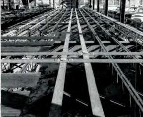
E/C Joists can be substituted directly for standard joists to provide as many electrical raceways as desired. The two header ducts, shown horizontally in the foreground, feed wires into the E/C Joists through the hand-holes in the center of the photograph.
