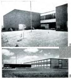
glass infill panels. The main level is raised six ft and cantilevered at either end over the basement wall. Overall dimensions of the building are 210 ft by 120 ft.
