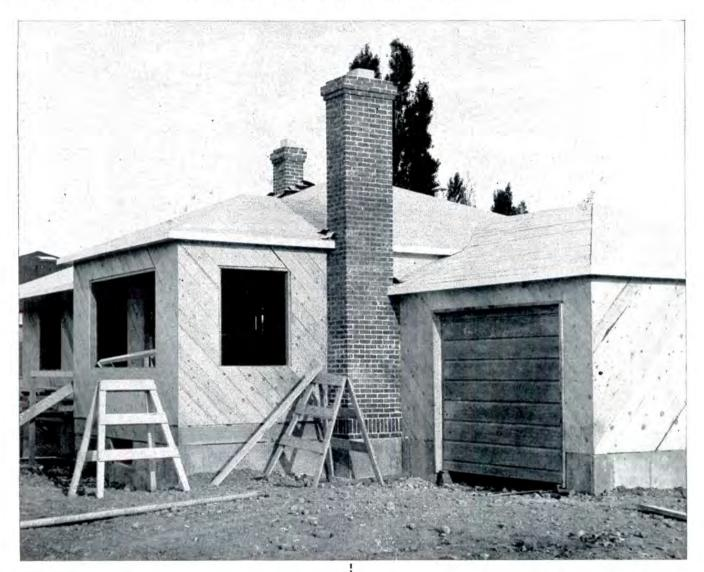
WHITE FIR makes a wise choice for sheathing. Not only does White Fir assure you a flat subsurface for siding, roofing and flooring, but it also contributes good insulating properties and adds overall structural strength to the building by providing stiffness. When you specify White Fir sheathing you are using a wood that nails easily and is light in weight to facilitate easy and economical handling on the job.
