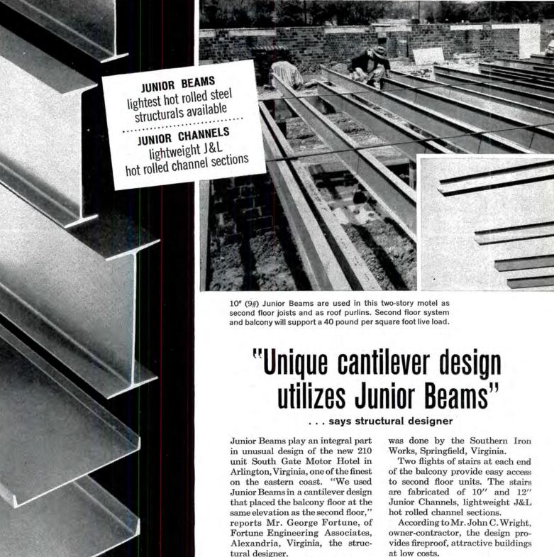
"This design eliminates steps from balcony into the units. The balcony is free of vertical supports," Mr. Fortune said. The three principal buildings utilize 170 tons of 10" (9#) Junior Beams, lightweight steel structurals made by Jones & Laughlin Steel Corporation. The Junior Beams are used as second floor joists and as roof purlins. Fabrication and erection at low costs.
