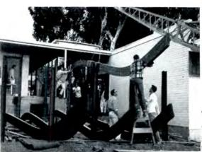
Nailed laminated beams form roof structure for seminar room being added to existing structure at CalPoly
