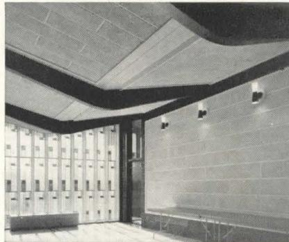
St. Mark's Episcopal Church, Columbus, Ohio. Decorative and functional use of Tectum for the two-slope, ceiling design and sidewall in the narthex of the church. Acoustical control plus decorative good looks. *Architect: Brooks & Coddington, Columbus. Contractor: Leo E. Ruisinger, Inc.*
