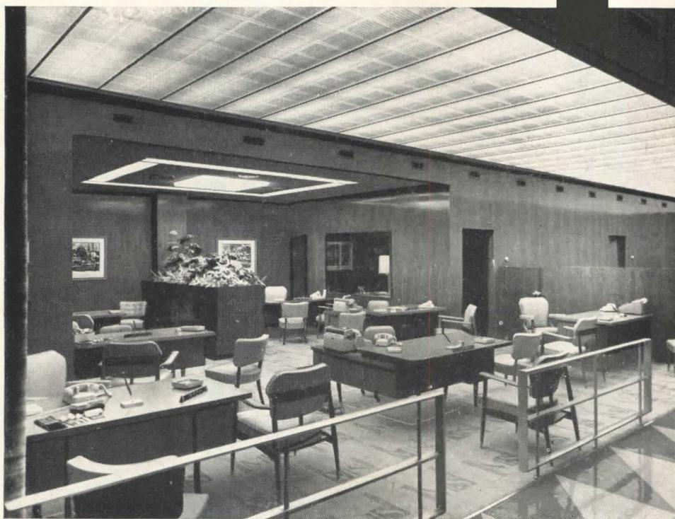
Even with Strato-Lux directly overhead, there are no bright spots, no reflections, in critical viewing areas. Acrylic plastic panels never discolor, can be slipped out one at a time and dipped in detergent for cleaning.
