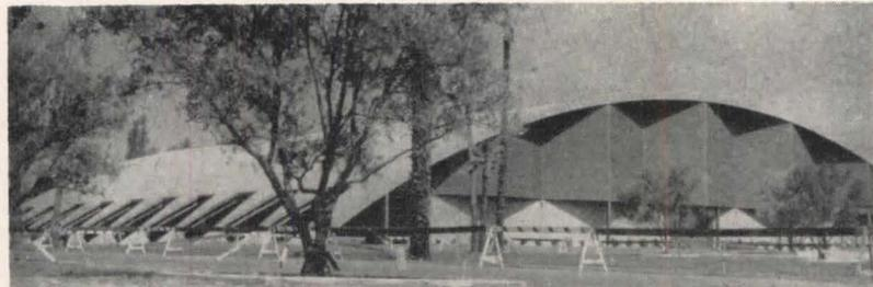
6. Though similar to the conventionally buttressed auditorium shown above, this exhibition hall represents an advance over it in that the need for buttress-type supports was eliminated by pulling the lamella barrel down almost to grade level and scalloping the frame between the low concrete piers. This proved to be doubly advantageous since the considerable reduction in the size of the buttresses cut expenses while the scalloping produced a pleasing esthetic effect
