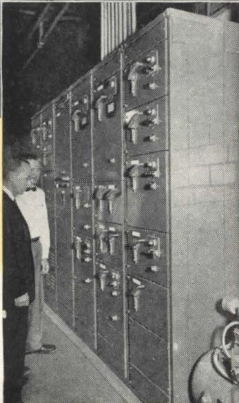
• This Square D control center in the Administration Building includes circuit breaker combination motor starters for the heat pump and air-handling equipment. Heat pump operation is automatically controlled through thermostats and programmed by clock system.
