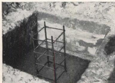
Vibroflotation stabilizes granular soil so effectively that excavations retain neat, vertical walls even after placement of reinforcing steel and pouring of concrete.
