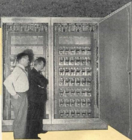
• Lighting (a high frequency system, 450 volts at 840 cps) in the Administration Building is controlled from this panel. Note space for future additions of Square D contactors as they're needed.
