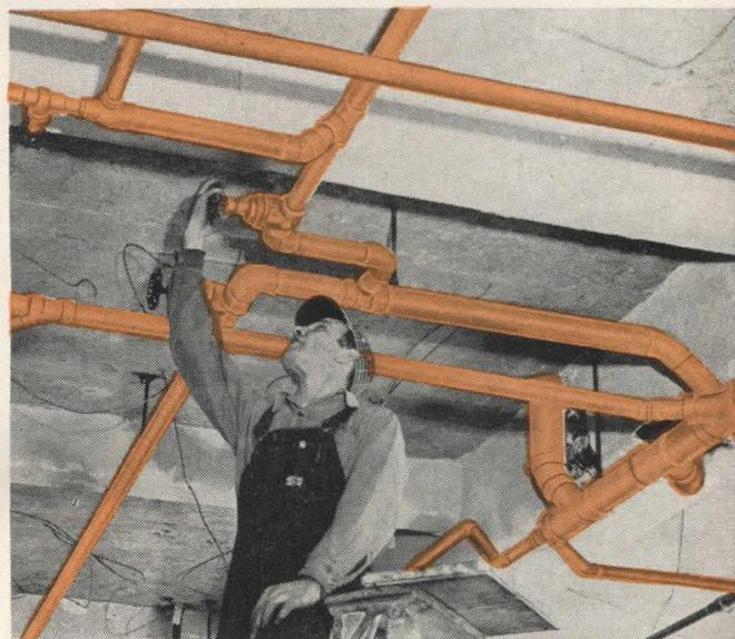
**TESTING A VALVE** on the hot-water supply system. Other copper tube lines in view are part of the sanitary drainage system, ranging in size from 1½ inches to 4 inches. Because connections are easily made, even in tight quarters, the lines can hug the ceiling.
