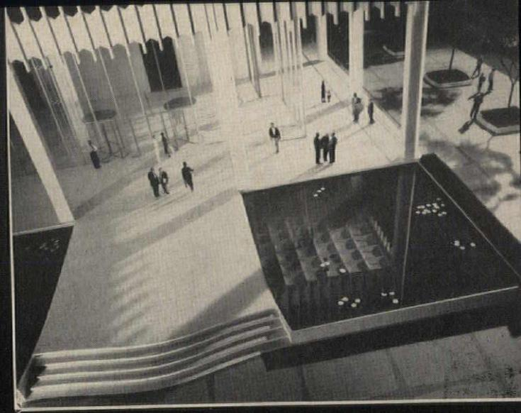
The mullions for the glass wall in the lobby will be pre-tensioned in order to achieve maximum lightness and delicacy—details are shown on this page. Pre-tensioning these 25 ft high members will reduce their required cross section by more than one half. The 4 ft 8 in. wide glass panels will angle in and out for interest and richness
