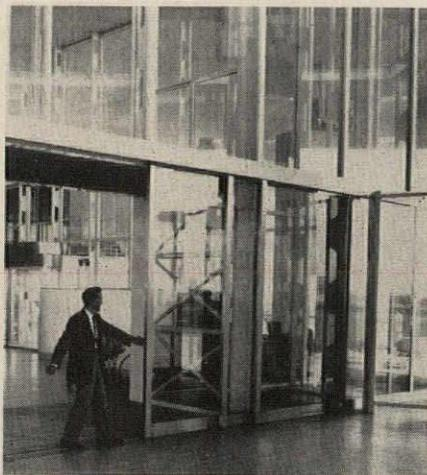
Left: Details of air entrance for Pan American Terminal. Front wind screen is shown top left. Side wind screen, supply grille and floor grating are in bottom photo. 15-ft sliding glass panels to close air entrance stack three deep at either side (top right)
