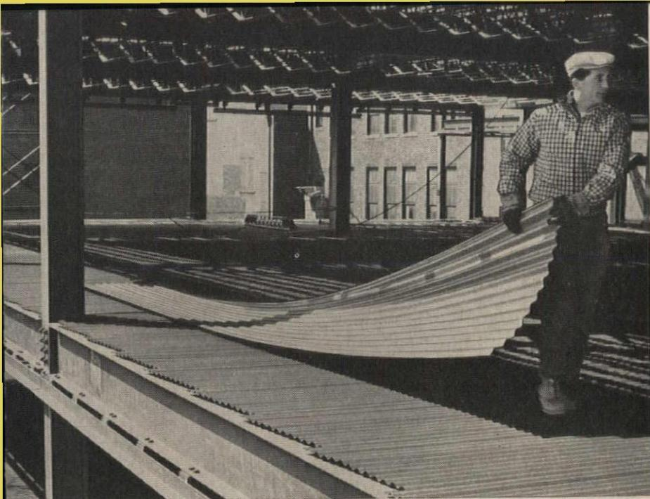
Extra-long lengths of coated Fab-Form, 27 feet, 3 inches, were specially commended by job superintendent on Looman Building job. "Fab-Form's extra-long length and wider width certainly helped to get these floors and roof poured faster," he declared. "I'm convinced the red oxide finish has better corrosion resistance than other coated sheet material."
