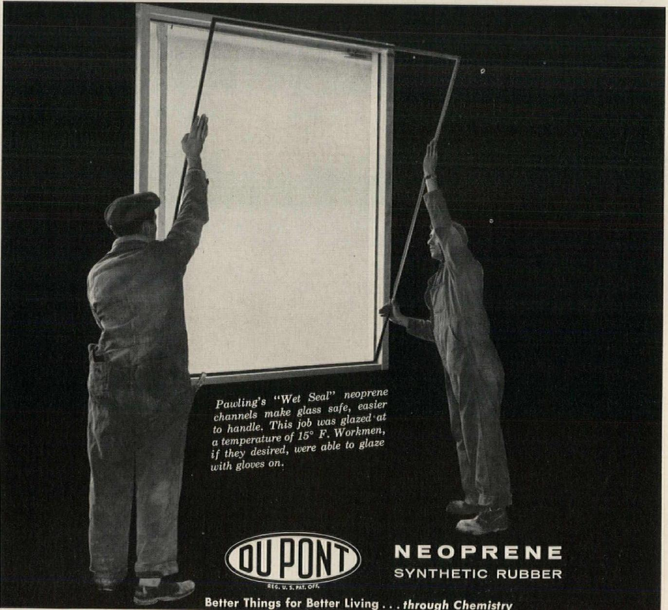
*Pawling's "Wet Seal" neoprene channels make glass safe, easier to handle. This job was glazed at a temperature of 15° F. Workmen, if they desired, were able to glaze with gloves on.*
