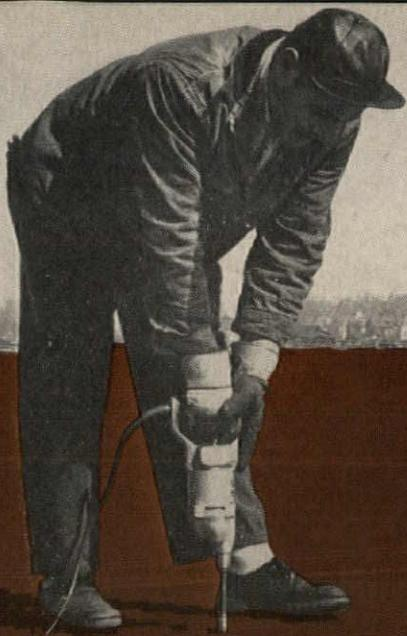
Coated Fab-Form's red oxide coating shields the base steel from corrosive elements in concrete. Here, on the roof of Looman Associates Office Building in Trenton, N. J., coated Fab-Form was installed by a four-man crew in just one day.
