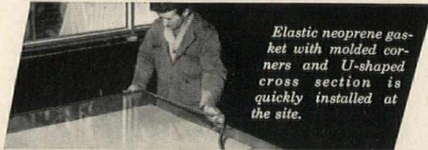
*Elastic neoprene gasket with molded corners and U-shaped cross section is quickly installed at the site.*
