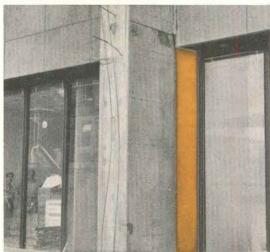
UPRIGHT CONCRETE GIRDER before covering with bronze "skin." The Revere Muntz Metal used was in thicknesses of ½" and 3/16", ranging up to 40" in width by 11' 11" in length.
