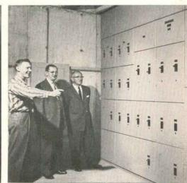
A. J. Eversmann, Maintenance Superintendent of WAVE, inspects the modern and compact Westinghouse building-type switchboard with R. A. Schlaug and M. D. Bornstein, both of Bornstein Electric Company. Westinghouse AB De-ion<sup>®</sup> circuit breakers distribute and protect all power circuits in the studio. Provision is made to install additional breakers when required in the future.
