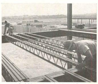
Steel joists arrive at the job site fully fabricated, ready for immediate placing.
