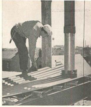
**Precision-manufactured**, Fab-Form easily fits around obstructions such as columns and pipes. Installation was easier and faster because corrugations line up precisely on end laps.
