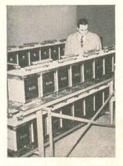
**Emergency power source** Powerful Exide Batteries can handle lighting loads for entire buildings. Long service life up to 25 years is common.
