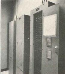
Westinghouse Type NA1B panelboards are used for distribution of the many lighting circuits in the studio. These circuit breaker panels protect circuits against overloads and short circuits.
