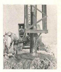
Vibroflot machine in action. Each compaction consumed 3 or 4 tons of sand.
