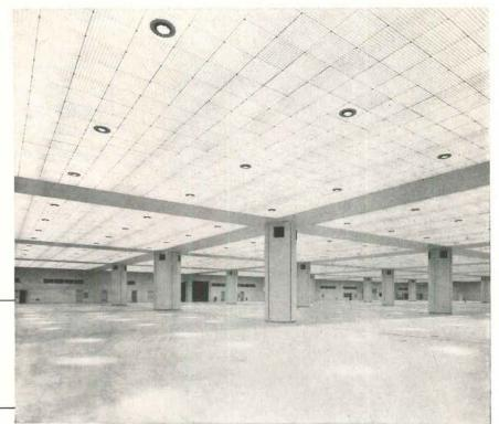
Sylvania's louvered ceiling provides 135 footcandles of general lighting for over 100,000 square feet of display area. Complete system consists of outrigger-type fixtures with eight 75-watt Instant Start lamps installed in a grid arrangement.
