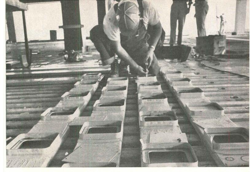
Spang Headerduct will feed electric, telephone and intercom wiring into floor cells on 28 of the 32 floors at First City National Bank Building, Houston, Texas. This will provide service wherever it's needed and permit speedy changes to meet any future requirements.
