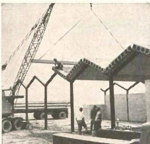
New 8" x 16" Hi-Stress units are fully pre-stressed slabs ( $f_s$  175,000 psi) cast in steel forms, with stress-relieved strands tensioned before concrete is poured. Appearance is similar to standard Flexicore slabs which use pretensioned intermediate grade steel bars.
