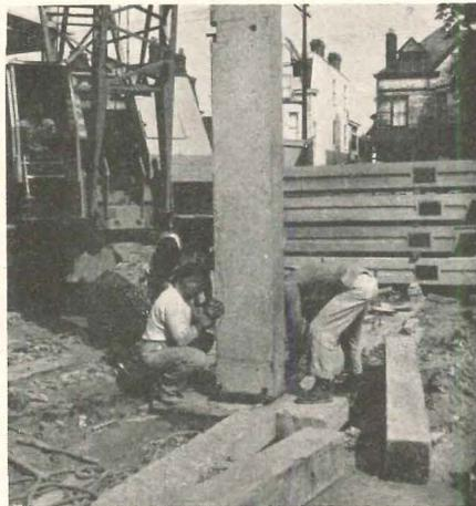
Precast columns are precision plumbed by bolting to steel plates set in the pile caps. Columns and ordinary reinforced slabs are precast on a vacant lot near the site
