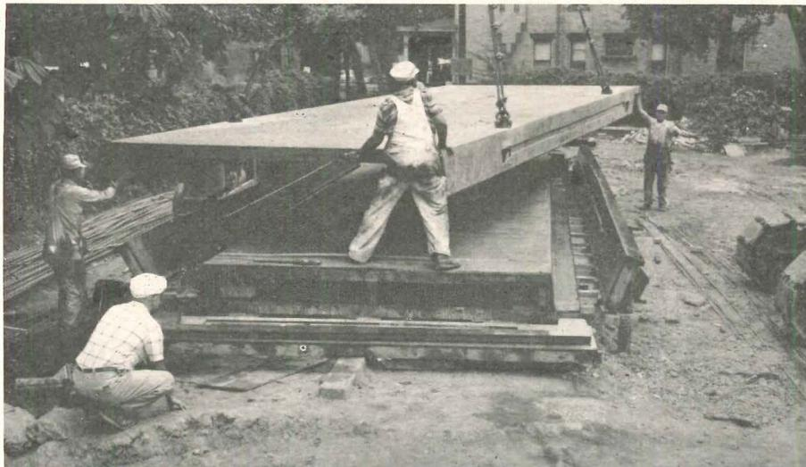
between slabs were simply filled in for required wind bracing after the mechanicals were installed.
