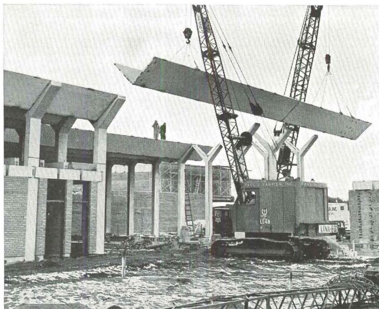
The folded plates for the cafeteria roof are 5'3" wide, 2 1/2" thick. Along the length of the building they make three spans of 60, 48 and 60 feet, with an 8' overhang at each end.
