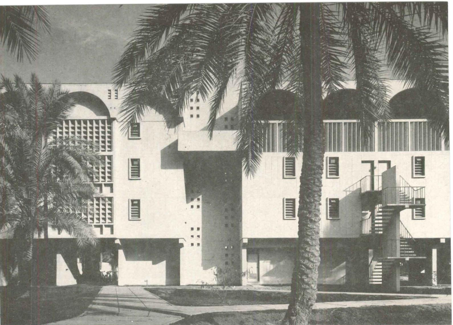
Staff housing. Double roof for protection against heat is formed by a series of high vaults under a flat tile roof. Air passes between the two roofs by means of louvers between each pair of vaults
