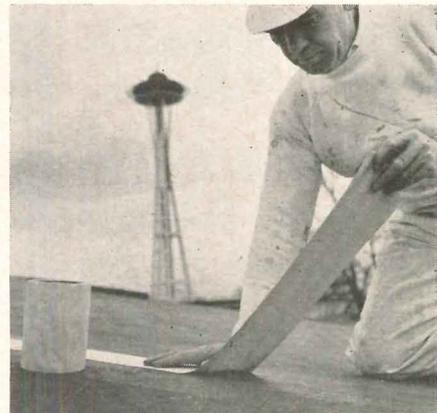
prevents seepage into joints of the vinyl-coating material used as a base waterproofing material. The tape's high tensile strength and tear resistance permits expansion and contraction due to temperature changes. *Permacel, New Brunswick, N. J.*
