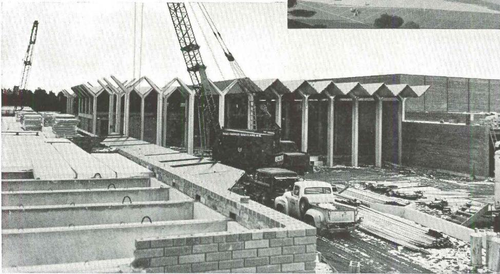
Folded concrete plates supported by 25' high Y columns form the cafeteria roof. At lower left are 2' x 4' lightweight roof slabs on prestressed joists. The roof slabs provide insulation and an attractive acoustical ceiling. All concrete roofing units are left exposed to inside view.
