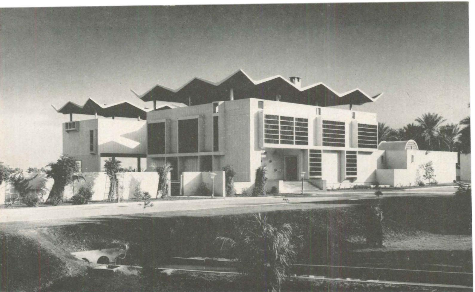
Ambassador's residence. It is protected from the sun by a hyperbolic paraboloidal parasol, which forms a reflecting sun shade and allows free air circulation below. Servants wing to right of photograph
