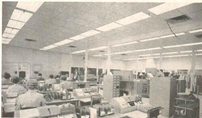
Fig. 7. Office lighted with twin aluminum troffers using 8-ft, 1500 ma lamps to provide 125 fc
