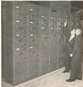
This motor control center, one of many supplied by Square D, contains Size 1 through Size 5 combination starters for control of exhaust fans, boiler feed pumps and condenser pumps. Ronald Martinec, Estimating Engineer for the electrical contractor, inspects this installation with Bob Kunz, Square D Field Engineer.
