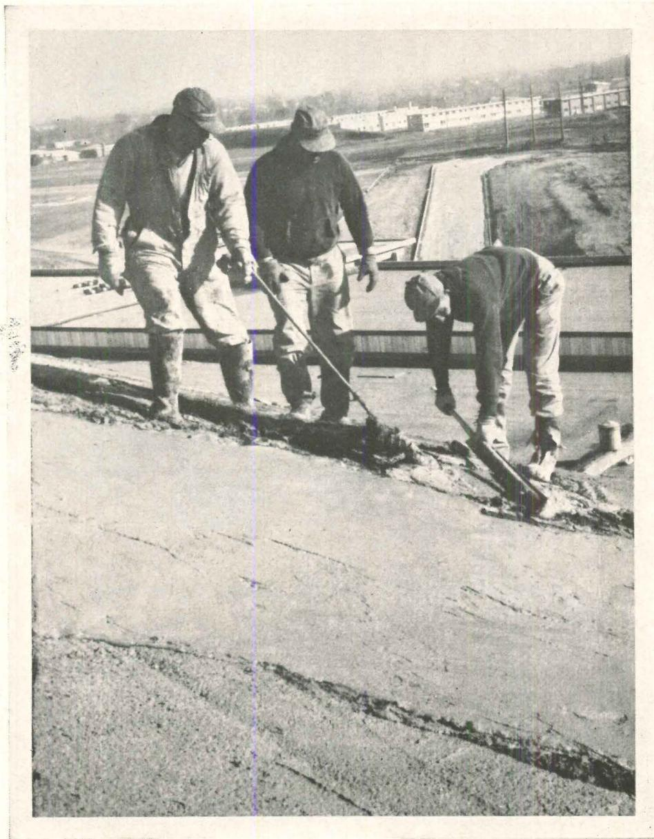
The application of **Zonolite** insulating concrete roof decks is as specified, *exactly*
