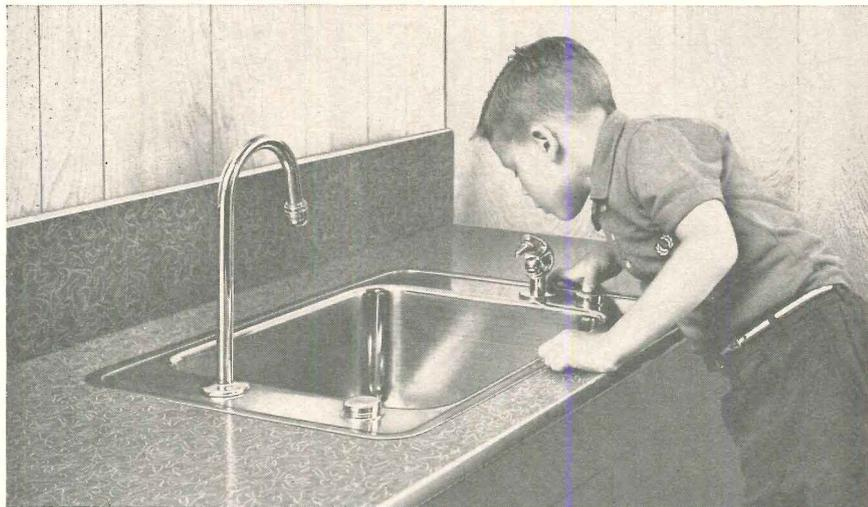
*This is Haws Model 2284 in stainless steel*—featuring the new Haws push-button valves that send vandalism worries down the drain! Slow-closing valves work smoothly under slight pressure: can't be jammed or pried. And the gooseneck is extra-heavy  $\frac{3}{8}$ " brass pipe: even *you* can't bend it! Same valves available on all Haws receptors, including enameled iron. Ask for the specs: write for details on Haws push-button valve.
