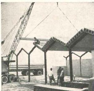
New 8" x 16" Hi-Stress units are fully pre-stressed slabs ( $f_{s1}$  175,000 psi) cast in steel forms, with stress-relieved strands tensioned before concrete is poured. Appearance is similar to standard Flexicore slabs which use pretensioned intermediate grade steel bars.
