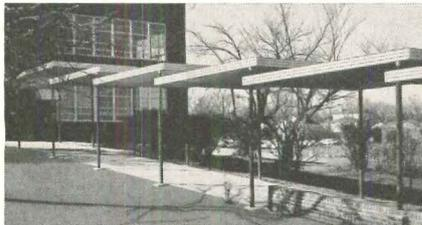
How's this for design versatility: You can select from six different types of facia, from a slim 4½" straight face to a big 11½" high facia with a bevelled extender to give a cornice effect. All facias are slotted to retain color trim aluminum strips in an almost unlimited range of color combinations.
