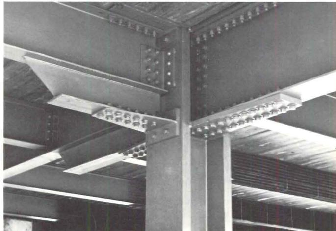
Close-up of column connection illustrates type of welded tees which were lab tested. A373 steel was used, with stress-relieved full butt welds. The bolts were extra-high-strength (140,000 psi minimum tensile strength).
