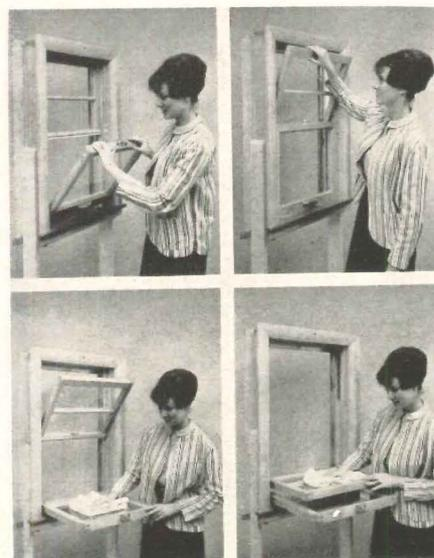
installed on any wood window sash without disturbing the frame. When closed the window can be operated or locked in the regular way. *Kaywood Windowware Corp., Box 187, Kalamazoo, Mich.*
