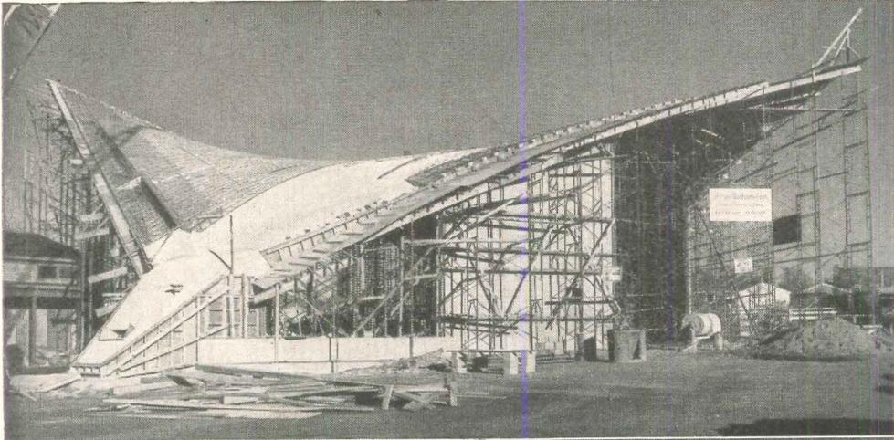
In the photo above, the portion of the shell with light-weight concrete is to the left of the abutment. To the right—the portion with the regular concrete (see diagram below). After shell was complete and concrete had attained 3000 psi compressive strength, it was post-tensioned both longitudinally and transversely. Below-grade tie beam between the abutments was also post-tensioned. Rigid insulation serves as the surface of the shell, thus becoming an integral part of the shell.
