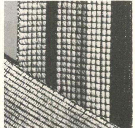
shown in picture, have a double face with striped wool on one side and asbestos-glass fiber on the other. When sun is strong, the louvers can be shut so only the sun-resistant asbestos-glass is exposed to the sun. *Verti-Color Blinds, Inc., 64 E. 55 St., New York 22, N.Y.*
