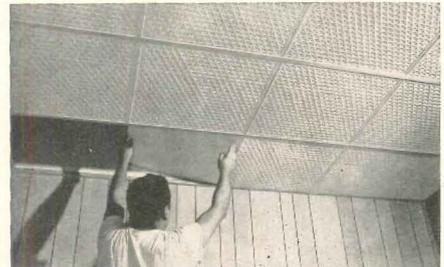
ranging from one to eight inches. They have a lap edge and may be installed by stapling, nailing or gluing. *United Progress Co., 54-60 Dott Ave., Albany, N.Y.*
