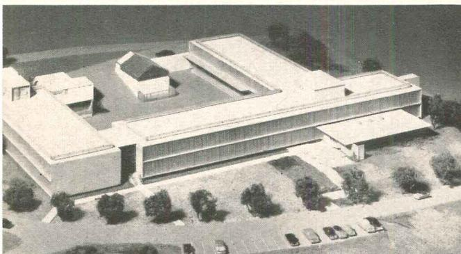
**V NUCLEAR MEDICINE BUILDING** at a Calif. university. Continuous way flat slabs, 9-in. thick are post-tensioned with 838 tendon assemblies Ryerson. Column spacing—about 25 ft. Architects & Engrs.: Neptune & mas & Assoc., Pasadena. Gen. Contractor: James I. Barnes Construction Santa Monica. Lifting: Vagtborg Lift-Slab Corp., Los Angeles.
