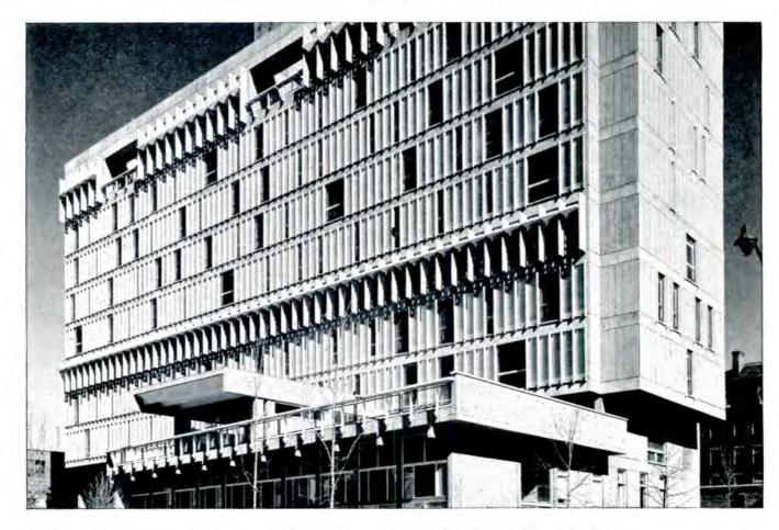
Freedom in fenestration has been carried forward a giant step by Architects Sert, Jackson and Gourley in Holyoke Center. The triple function of providing light, ventilation and view has been re-examined and applied room by room to serve human needs. The result is better use of light within and unusual exterior interest.
