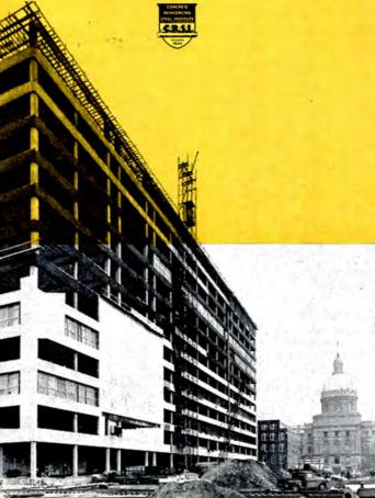
■ In the construction of this new Indiana State Office Building, a monolithic reinforced concrete frame helped maintain minimum costs. Other construction materials had been considered, but by actual cost comparison—based upon building height and width—monolithic reinforced concrete frame and one-way joist floors proved to be the most economical.
