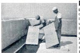
Nothing but FOAMGLAS Roof Insulation gives a building the constant insulating value that results from an inorganic, cellular glass composition. It just can't absorb moisture. And,
