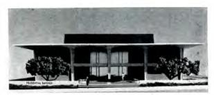
BRANCH BANK: This two-story building for Prudential Savings and Loan Company in Alhambra, Calif., is of concrete and brick filler panels. Structural concrete columns, handsomely shaped, support a flat plate concrete roof; inside, the ceiling of the banking room is slightly vaulted, and is daylighted by a large central skylight. A mezzanine work area around three sides of the banking room provides public meeting facilities and office space. Architects: Ladd & Kelsey
