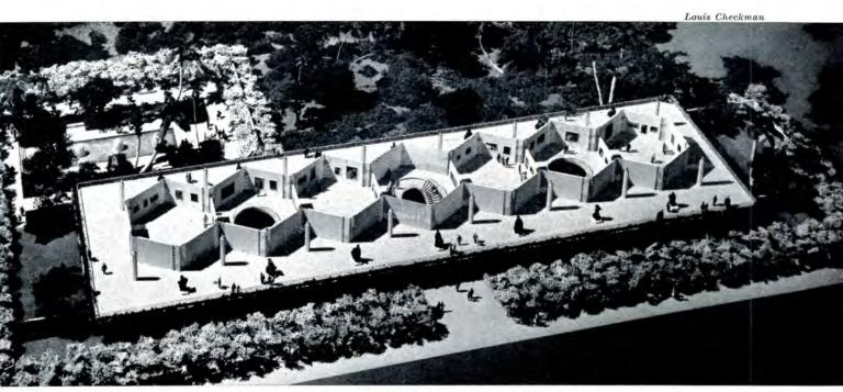
The climate is so mild in Ponce that air conditioning is not necessary. The galleries are all open to the air at each hexagonal point. In case of hurricane sliding mahogany panels will close in the area defined by hexagonals
