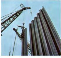
Just a stone's throw from Constitution Plaza, contractors pound home Bethlehem Steel sheet piling for substructures along I-84. Also on the job: Bethlehem H-piling, bracing, concrete reinforcing bars, and paving steels.
