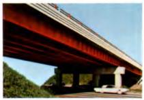
The viaducts, grade crossings, and interchange bridges on I-84 and I-91 are steel. Bethlehem is supplying thousands of tons of structural shapes and plates to the fabricators, The Standard Structural Steel Company and Trans-United Industries Inc., City Iron Works Division, both local firms.
