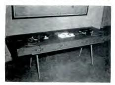
classroom use, has monaural and stereo four speed turntables and a tape recorder. There are three circuits each with twelve headphone jacks for individual listening. The equipment can be used for public address, and the teacher can record on tape without being heard by students. The table is 32 by 92 in. The Perry Co., Box 7187, Waco, Tex.
