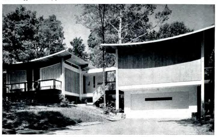
Wood bests any level, as demonstrated in this modern home topped with twin oriental-flared roofs grace-fully supported by full-length laminated beams, double-posts bolted together, and siding solidly planked from corner to corner. This structure of striking simplicity was designed by Jay Fleishman, architect.
