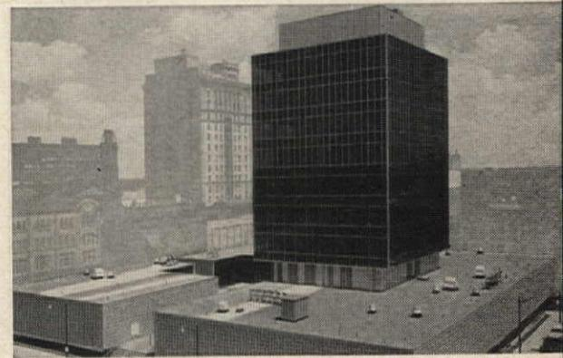
**THE NEW CANTON CITY HALL, CANTON, OHIO**, takes full advantage of Republic's ENDURO® Stainless Steel: in mullions, column sheathing, curtain wall panels, rooftop equipment, doors, windows, elevator interiors, soffits, fasciae, and curtain wall back-up members. Need for painting was eliminated, cleaning reduced, maintenance minimized. For further information contact your nearest Republic representative or check Sweet's.
