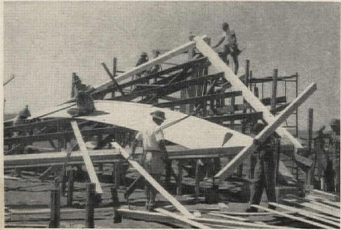
Second layer of boards is nailed to first in concave curve
