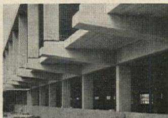
Lateral beams at second floor cantilever 7'-3".
