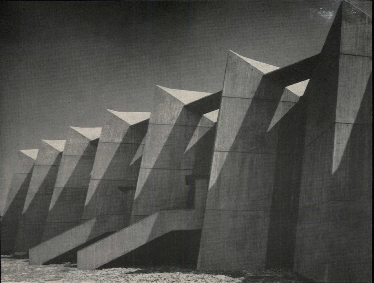
Tensile beams connect all unit arches together, pulling them toward the rear of the building
