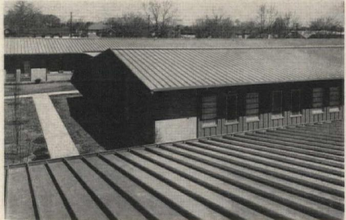
num with a uniformly deposited coating thickness of approximately .002 in. per side—twice the thickness of a commercial hot dipped zinc-coated steel. General surface corrosion resistance of the coating in normal atmospheric exposure is similar to 1,100 aluminum.
