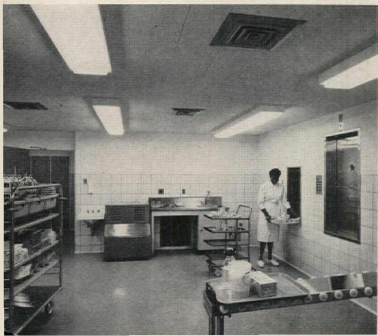
tion, an auxiliary dumbwaiter connects all levels, primarily to take nourishment from the central kitchen to the patient floors; it may also be used to return clean supply trays and tote boxes from the clean supply cores on each floor to the dispatch center issue area.
