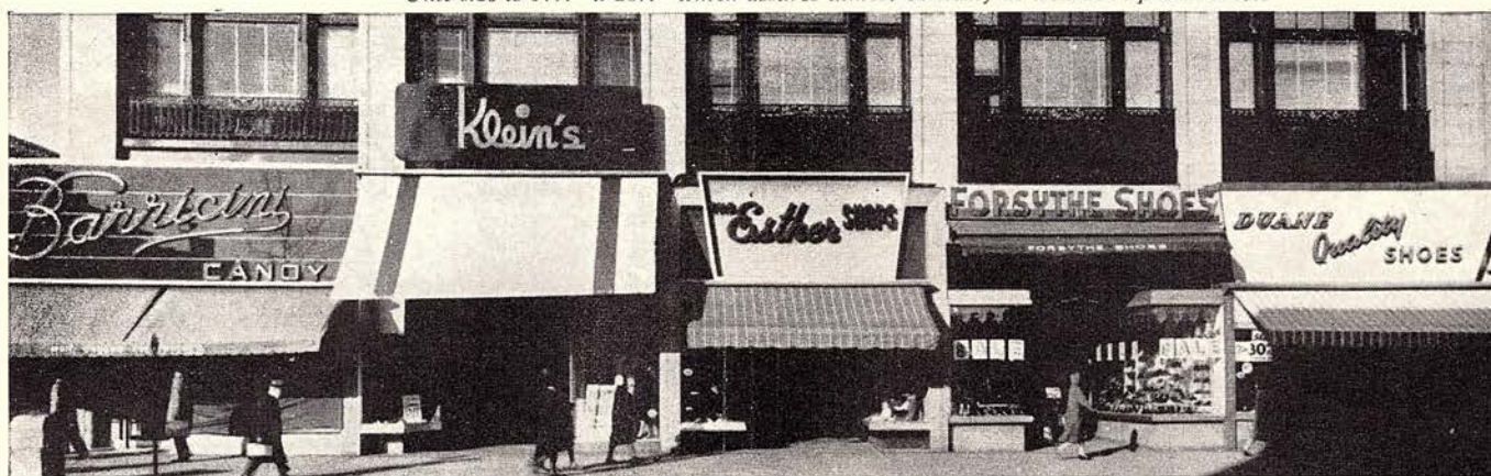
Hahn Store, Washington, D.C. Edmund W. Dreyfuss & Associates, architects. Standard Art Marble & Tile Co., contractor. For this enlarged and modernized store the architect created a distinctive white facade by specifying the repetitive use of CV Durathin Design No. CVD-13X. Wherever a deeper relief is desired as in this instance, the CV Durathin Design can be reproduced in thicknesses up to 1½" Unit size is 17¾" x 23¾" which assures utmost economy as well as impressiveness.
