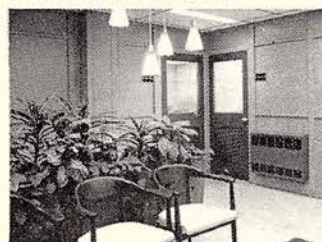
Convection heater in reception room.
