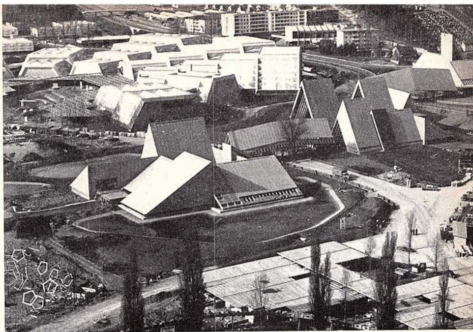
Above: Middle ground, the Swiss Way. Background, Industry and Crafts, a fan-shaped pavilion of tubular steel construction covered with canvas. Below: Foreground, the Joy of Living, with facades of wood and roofs of plastic. Background, Culture, Science and Art, steel columns support asbestos-concrete roofing elements and are faced with pressed-wood panels, laminated white plastic sheets and transparent polyester sheets. Cubic sections are grouped around a court containing 20 pieces of sculpture, cast in aluminum and gilded
