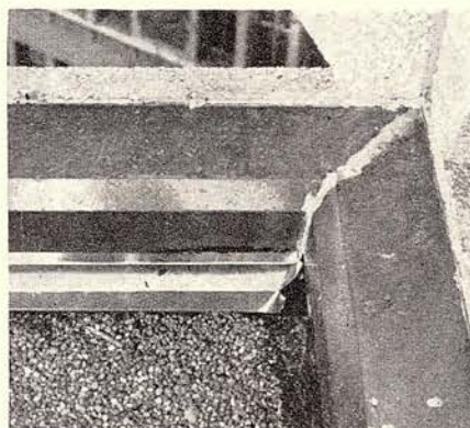
Corner details for building at top. Counterflashing is hooked to base flashing ( right ). Prefabbed corner sections have been caulked to insure against leakage. Flashing here is copper; anodized aluminum and galvanized steel are also used
