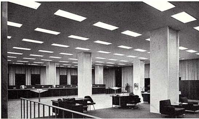
Sunbeam Lighting's VISIONAIRE-5 air-handling luminaires light bank.
