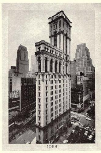
When its 3700-ton steel framework was erected in 1904 by American Bridge, the Times Tower was the tallest building in New York. Plenty of later buildings dwarfed the 24-story skyscraper, but few ever matched the fame the Times Tower gained from the electric news sign that flashed around its circumference and was seen daily by a million and a half people.
