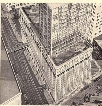
This building has two levels of below-grade parking, nine levels of sloped-floor parking above ground-level retail space. The parking decks are served by a ramp that winds around the building, sometimes (at left) outside the building line. At top: two levels of office space, an apartment tower
