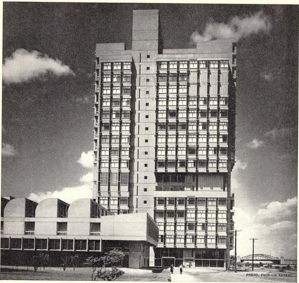
The 18-story building houses the Law and Education Departments. It rests on a floating foundation 13' thick, 60' x 140'. Window frames are precast concrete and provide space for vertical ventilating panels made of colored metal. Smaller building in left foreground is the Pappas Law Library.
