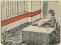
Reception Areas Chromalox Electric Sill Line and Baseboard Units are available in a wide range of models and heating capacities. Sill lines are usually mounted under windows, baseboards at floor level for continuous wallto-wall heating in offices, reception areas, corridors and similar applications.
