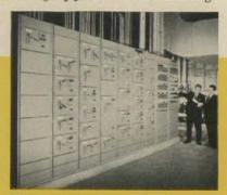
This Square D motor control center provides remote operation of the building's ventilating and heating system. Ward Ruske, Square D Field Engineer, and Carroll Burnett, Project Engineer for Super-Hatfield, check out a special Square D panel that indicates visually which motors are operating. Other control centers serve other areas.
