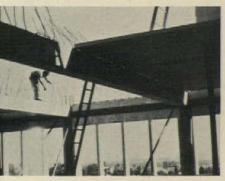
After exterior wall panels were set, columns were poured. Next, beams spanning 36 ft were placed between exterior panels and the poured-inplace core, or, as in the photo, an interior column. By using a structural core, only three interior columns were required. Job efficiency was increased by simplicity of the connections. Steel reinforcement projecting from wall panels, beams and slabs ties them to the topping. Total construction time for erecting the nine-story structure was four months.
