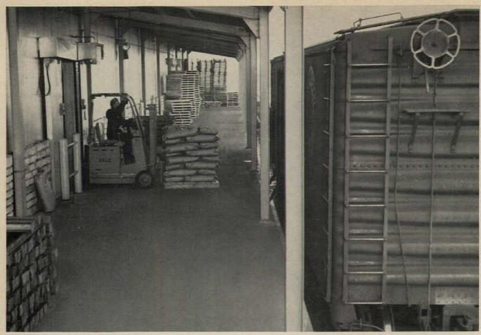
Fast, automatic operation of Electroglide Mark II doors on warehouse loading dock permit rapid transfer of frozen foods to refrigerated cars.
