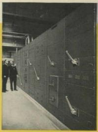
Earl Towery, Structural Engineer for the architect, and Bob Colby, Field Super-intendent for the electrical contractor, inspect the Square D main service switchgear. Square D I-Line feeder duct distributes 15,000 amps of power from this point to all other parts of the building.
