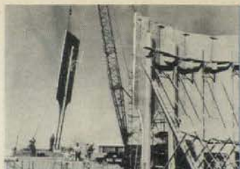
Prestressed concrete single tees swing into place
