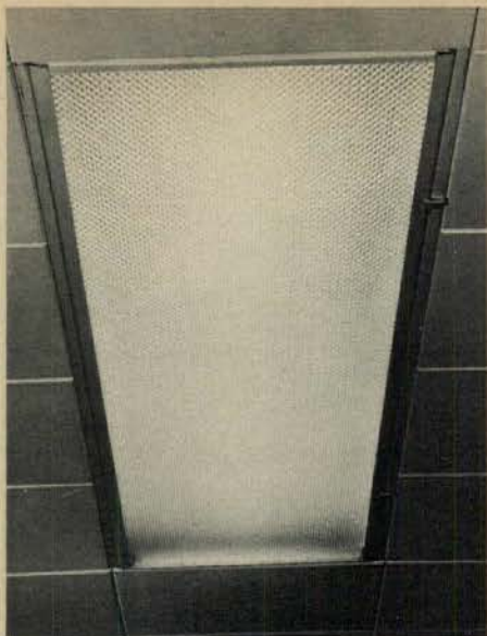
Small hexagonal prisms in glass panels direct light toward work surface, away from eyes.
