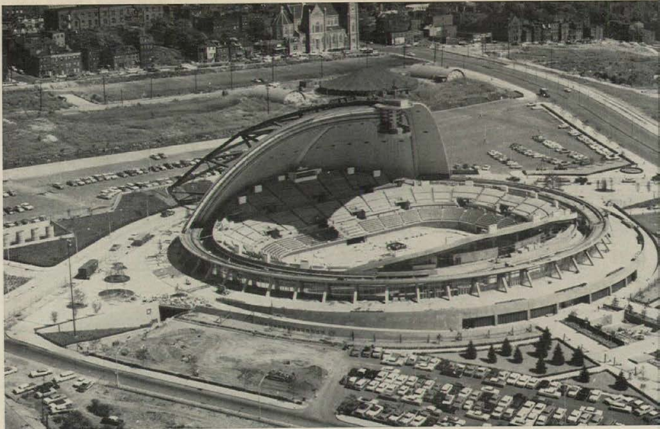
In 1960, Pittsburgh's 415-ft. clear span dome was the biggest in America. (And it's retractable, no less.)
