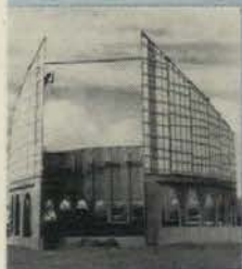
Prestressed concrete single tees swing into place
