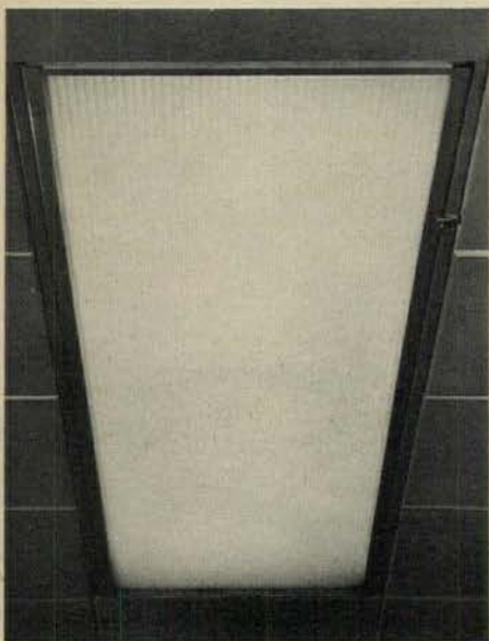
Opal diffusing panels obtain light diffusion through glass composition, not a pigment.
