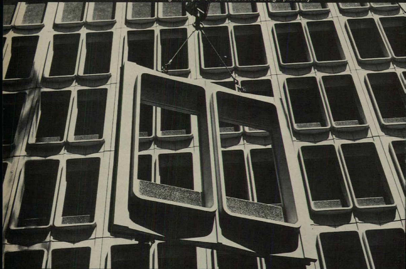
Schokbeton precast concrete double-window curtain wall unit, Sir George Williams University, Montreal, Canada Architect: Ross, Fish, Duchesnes & Barrett. Schokbeton by Schokbeton Quebec, Inc.
