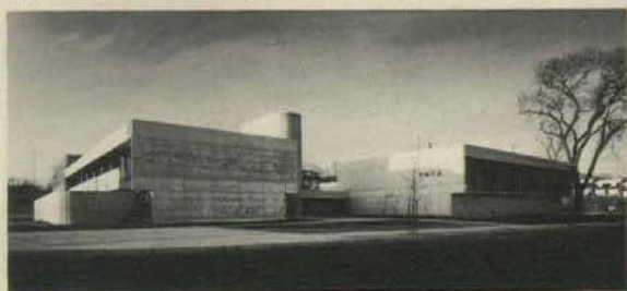
On the street side, the reinforced concrete structure is essentially closed on the pedestrian level; but the second level and the rooms open to the interior courts have large glass areas. Both plastic-coated and random vertical-board forms were used to vary the texture of the unfinished concrete.
