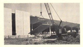
18-ton wall panels were tilted and positioned in as little as 2 hours each with a special telescoping steel strongback devised by the contractor. This was mounted to the panel's upper face and hooked to a crane. The strongback carried two removable jacks with wheels that reached beyond the inner (base) end of the panel, allowing it to roll outward as it was lifted. Once the panel cleared the roof, the wheels were dropped and the panel was turned 180 degrees and fitted to the wall.
