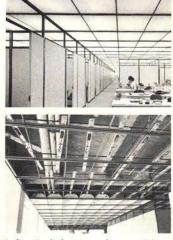
A first in lighting-cooling-partitioning flexibility was the ceiling of SOM's Union Carbide Building, for which Syska & Hennessy were consulting mechanical and electrical engineers. This system of continuous fixtures marked by a grid which functions for both air supply and partition anchoring was fully described in the February 1960 RECORD
