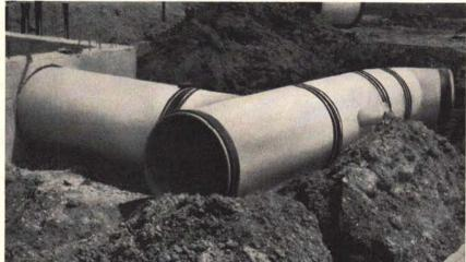
For the architect, a Johns-Manville TRANSITE\* air duct system below slab means minimum interference with structural elements. Ceilings can be higher. Glass areas can be more extensive. Building silhouettes can be lower. Furred ceilings and beam construction can be forgotten.
