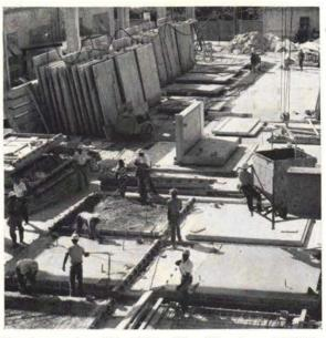
Panels vary from 9' x 12' to 17' x 12' and are 6" thick. Chattahoochee stone and special sand were used as aggregates to produce shades of brown and tan. Carved sections of foamed polystyrene were laid in 6" steel forms and concrete with the necessary reinforcing steel placed over them. When moulds are stripped, the polystyrene is destroyed.
