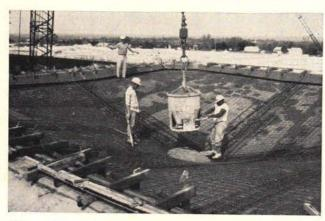
Through use of 4,000 psi high-early-strength concrete, shells were concreted at a 2-per-day rate. Before form removal, specifications required a strength of 3,200 psi, which occurred in 36 to 40 hours with the following mix proportions: Type III cement, 564 lb.; water, 267 lb.; sand, 1,300 lb.; 3/4-in. aggregate, 1,890 lb.; entrained air, 6 percent.
