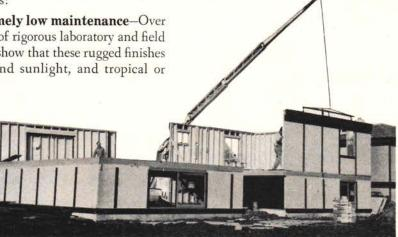
Wall section for this new house is lifted by boom crane and moved into position for installation. Interior wall is completed with foil-faced fiber insulation and ½ in. dry walls. Prefabricated walls are erected quickly and easily.
