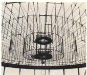
A great deal of engineering sophistication is built into the modern cable roof. In the example above loads are carried to the ground by a lightweight X-frame which also prevents bending in the compression ring when there are unbalanced loads. The Oakland-Alameda Coliseum by Skidmore, Owings & Merrill, San Francisco; roof consultant, Ammann & Whitney. Struts in the cable roof, left, together
