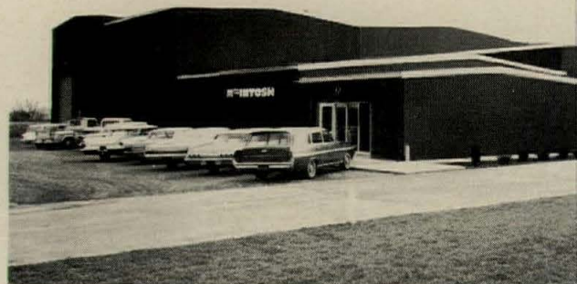
$13,000 SAVING: 32,000 sq. ft. stamping plant of McIntosh, Berne, Ind. Architect: C. E. Notzel, Detroit, Mich. Heating Engineer: Berne Electric Co., Berne, Ind. Contractor: David P. Construction Company, Warsaw, Ind.
