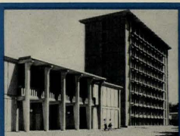
UNIVERSITY OF CALIFORNIA Davis, California Architect: Gardner A. Dailey, FAIA, & Associates Engineer: T. Y. Lin, Kulka, Yang & Associate
