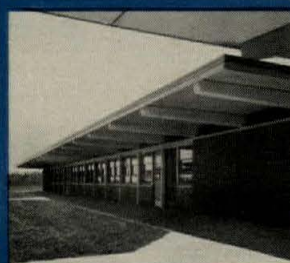
HENRICO HIGH SCHOOL Richmond, Virginia Architect: J. Henley Walker, Jr. AIA
