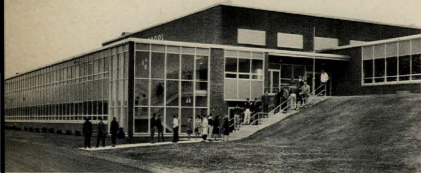
$63,000 SAVING: 675-student, 60,000 sq. ft. Hampshire High School, Romney, W. Va. Architect: Robert J. Bennett, Morgantown, W. Va. Engineer: Ballard & Mayfield, Canton, Ohio. Contractor: Baker & Coombs, Inc., Morgantown, W. Va.
