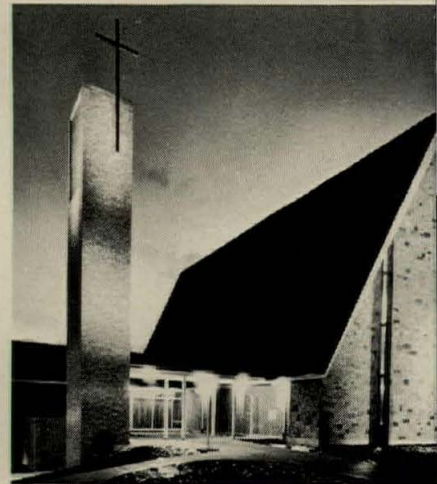
$10,000 SAVING: 18,500 sq. ft. Gloria Lutheran Church, Forestville, Conn. Architect: Jeter & Cook, Hartford, Conn. Engineer: James S. Minges & Associates. Contractor: Wadhams and May Co.
