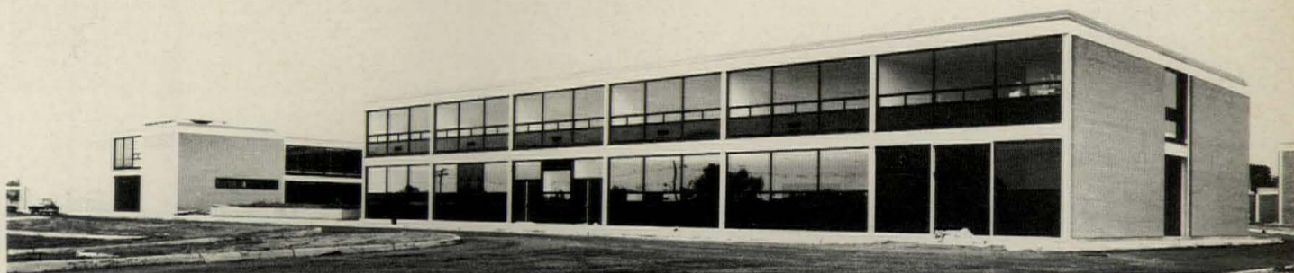
Monmouth Regional High School addition , New Shrewsbury, N.J. Architects: Kelly & Gruzen; contractor: Gumina Building & Construction Co.
