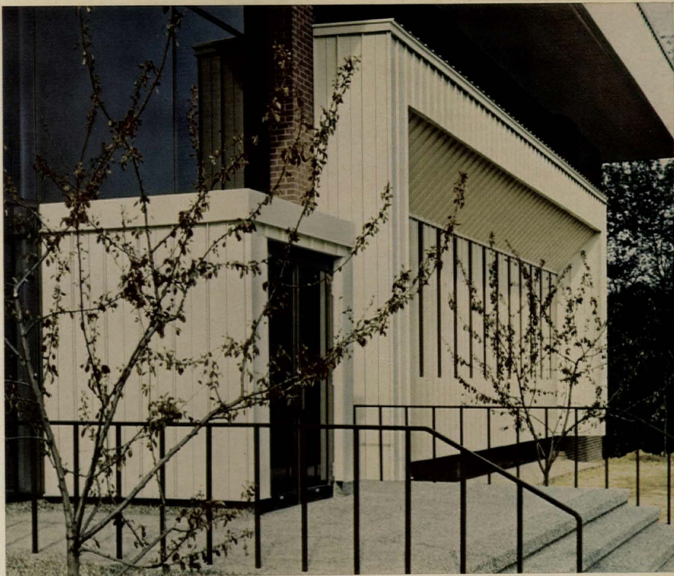
New office building of Elwin G. Smith & Co. Inc., Pittsburgh, Pa., has exterior metal protected with Fluropon † , made with Kynar 500.
