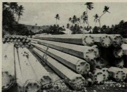
Prestressed beams for the ILIKAI Hotel addition made with MARACON by Prestressed Concrete, Honolulu, Hawaii. General Contractor — Pacific Construction Company, Ltd., Honolulu, Hawaii.
