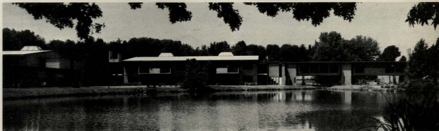
Meadow Lakes Village Presbyterian Homes , Hightstown, New Jersey. Architect: Richard J. Chorlton; contractor: Masset Building Company.
