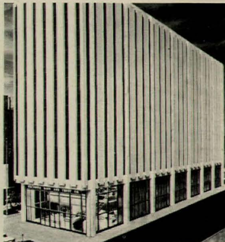
$13,700 SAVING: 120,000 sq. ft. Wachovia Bank and Trust Co. Building, Raleigh, N.C. Architect/Engineer: A.G. Odell & Associates, Charlotte, N.C. Contractor: T. A. Loving Co., Goldsboro, N. C.
