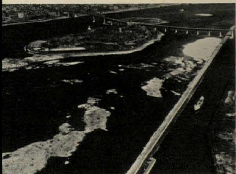
The site under construction, top, with the City of Montreal in the background, was created by land-fill from small islands, above.
