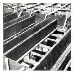
Gunnar I. Johnson, Minnesota contractor on the 4 story Science Hall at St. John's University, used a unique pan and joist construction shoring method to support 24" deep, 81/2" wide joists. Joists were 4' c.c., and shoring had to be held exactly to these dimensions.
