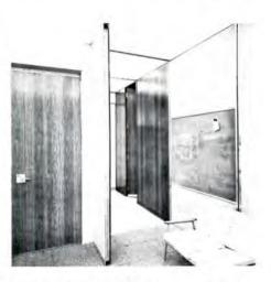
MOVABLE WALLS / A system that can be installed in schools, restaurants, offices and other heavy traffic public areas provides an acoustically-sealed flat wall that can be readily moved by custodial help to suit changing requirements. Mechanically expanded rubber shoes press against the floor and ceiling to close the opening. No floor track is required.
