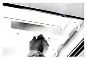
To change from a two-lamp to a four-lamp fixture it is necessary only to snap open the lens, shorten the special telescoping wiring channel, and unlock the wing bolts which hold the channel in the troffer. The entire channel, containing sockets, ballasts and wiring, is held by a chain while the workman unhooks wiring.
