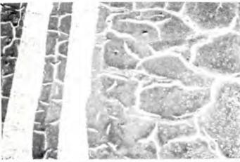
High temperatures (solar heat or too high kettle temperatures during application) can cause loss of volatile components in the bitumen, resulting in shrinkage of the bitumen and exposure of felts. This can be recognized by the pattern illustrated above. Then during winter weather, cold embrittlement cracks develop (shown below). The heat of summer turns these cracks into the familiar alligatored surface seen in the photo, right.
