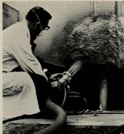
**INSULATION** / Two spray mixes (one for 2200 F and one good to 1350 F) go on at 600 lb/hr with no nozzle clogging and low rebound loss. Application technique permits rapid insulation of industrial equipment. Both mixes provide a laminate construction which permits varying of wall thicknesses. ■ The Babcock & Wilcox Company, Augusta, Georgia.
