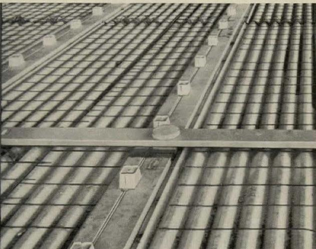
Factory-installed single, double or triple inserts can be spaced at any centering along cells to provide access to single, double or triple cells. Service fittings can then be installed at any desired location. Openings in inserts are designed to facilitate pulling large cables.
