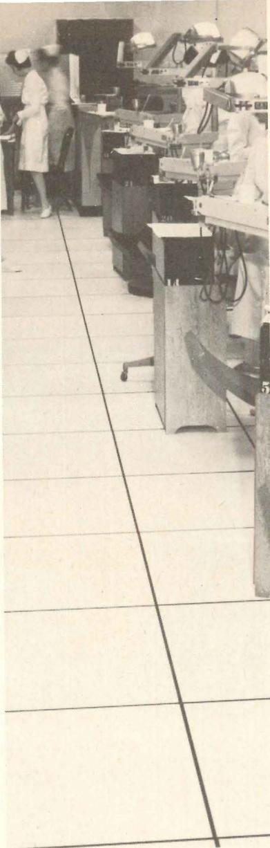
Now, see what it's done for a laboratory area. Electrical, water, gas, air, and drainage lines are completely concealed, yet completely accessible for repair or alterations. Lines can be brought up anywhere, even the middle of the room for full design freedom.
