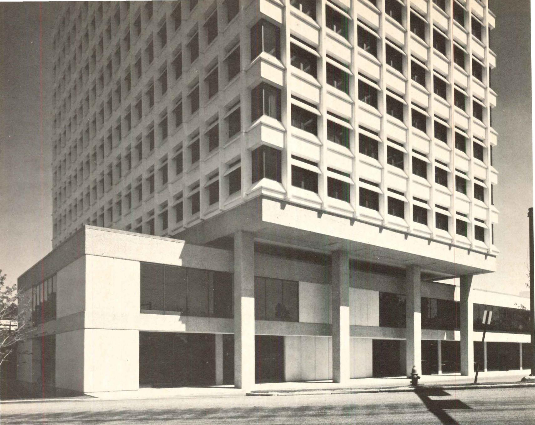
The 10-story rectangular tower is divided into three bays on the narrow side and six bays on the wide. Tucked beneath the front half is a two-story element with the main entrance lobby, shops and a restaurant on the second floor. Shown above is the building as it appears from the off-street parking area, approaching the lower level entrance.
