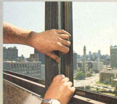
Butyl tape easily unrolls from roll, adheres quickly to window frame. Workers set large pane in place over tape for quick, weathertight seal.
