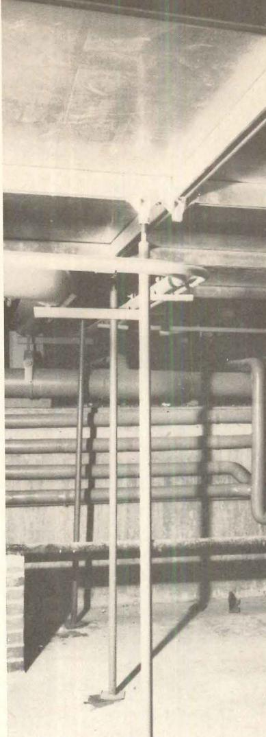
Lowered ceilings are a commonplace technique in renovation work. But here, they raised the floor. This avoids ripping out, provides an ultra-convenient place to run utilities. A simple way to even up different levels varying from inches to feet.
