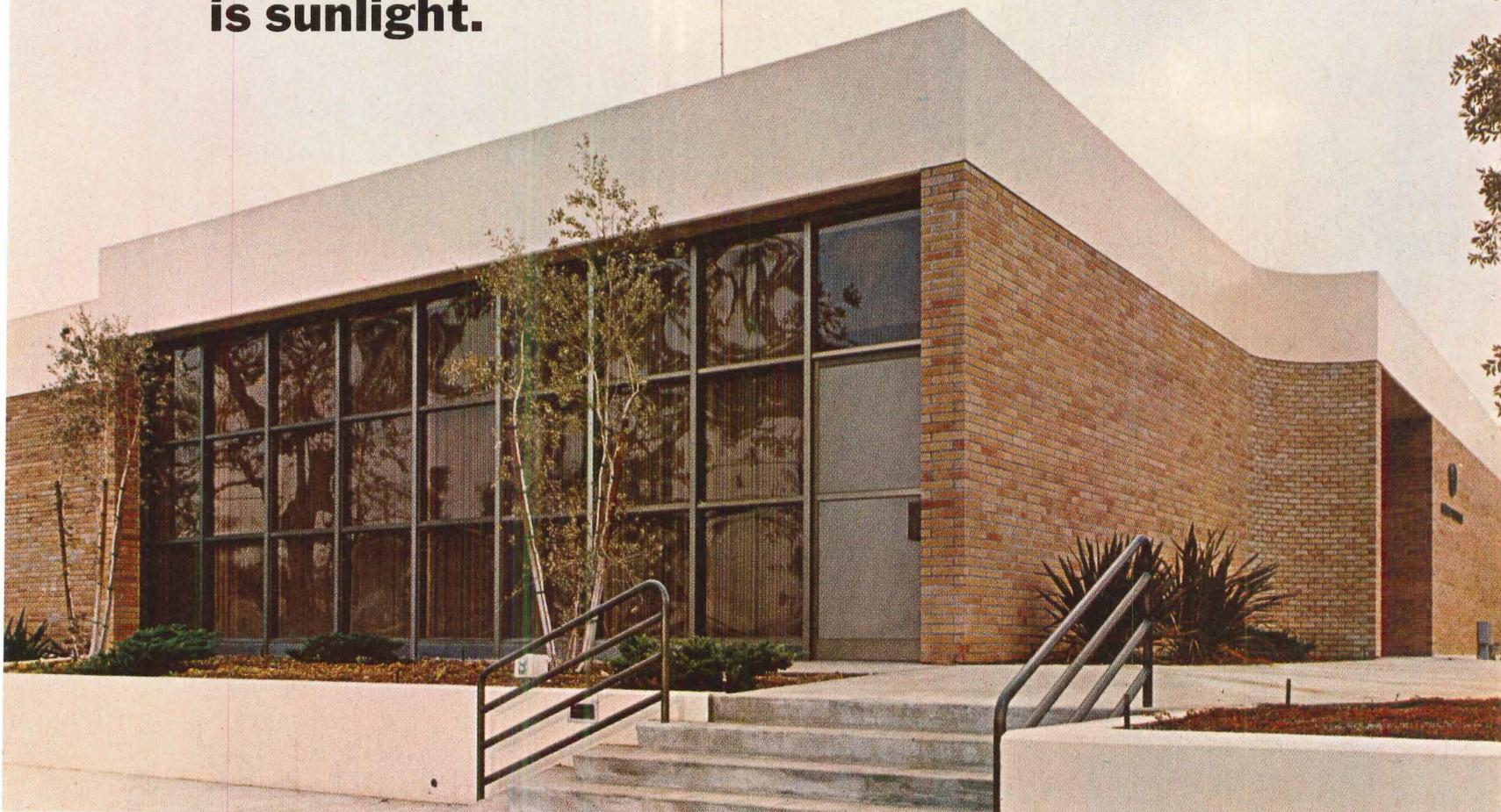
Companies that live in glass houses learn to take the breaks as they come. Not so with General Telephone Company of California. They are protecting complex communications equipment with unbreakable, solar tinted LEXAN SHEET for glazing. LEXAN just won't break. Thirty times tougher than cast acrylic, it shrugs off rocks, bricks, baseballs. It doesn't crack, chip or
