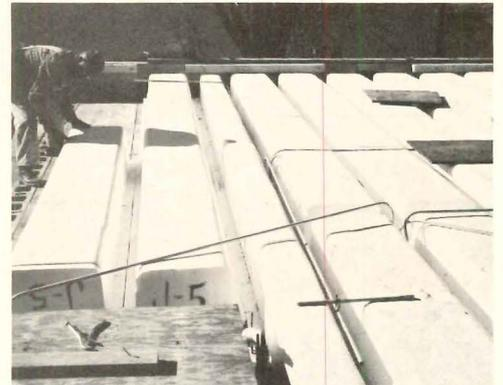
with the wind blowing the lightweight pans off trucks. If a piece of foam is broken off, however, it can be easily glued back in place.
