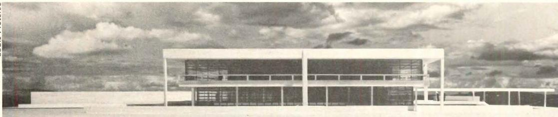
**Restaurant building** for University College Dublin, Belfield, Dublin, is sited in an artificial hollow that permits a three-story building with the main entrance on the middle floor. The building here, with projecting roof, is the first stage of a two-stage design to allow expansion. Architects: Michael Scott and Partners.
