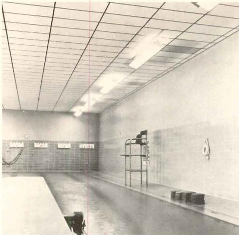
**SOUND CONTROL** / Glazed total ceramic acoustical panels are recommended for indoor swimming areas because they control noise and are dimensionally stable in high humidity. ■ The Celotex Corporation, Tampa, Florida. *Circle 300 on inquiry card*
