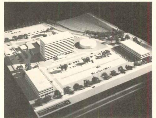
Etobicoke General Hospital in the north-western area of Metropolitan Toronto, planned for completion in 1970, is designed to accommodate an overhead monorail distribution system. An acute treatment hospital of 500 beds, it is master-planned to become, with the completion of future medical offices, extended care and educational facilities, a fully integrated health center.
