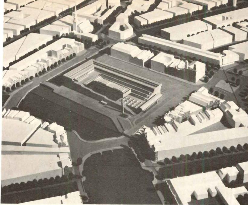
**Amsterdam City Hall** competition winner is this design by Austrian architect Wilhelm Holzbauer. The reinforced concrete structure—which is boldly skylighted—will have a brick veneer, and brick will be used extensively in the broad stepped-down terraces and river-
