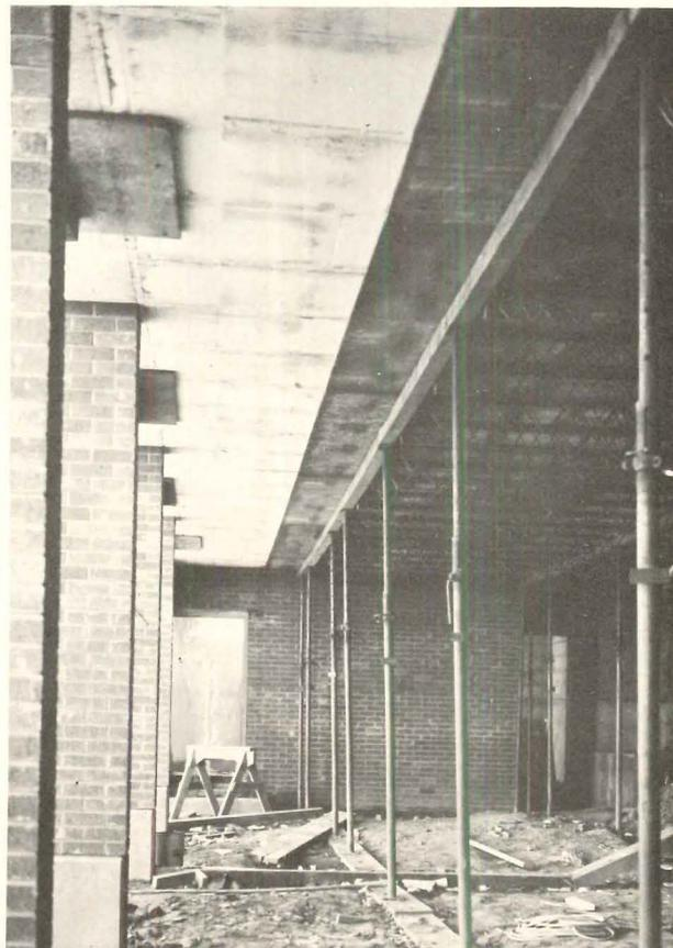
Shoring and plywood have been taken down in the vicinity of brick pilasters, showing how the pan ceiling looks prior to finishing. Cracks between the pans are bridged by the finishing material.
