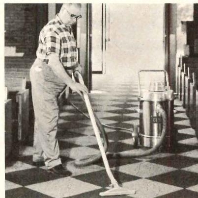
**MAINTENANCE.** Heugatile's dense pile keeps dirt surfaced for easy removal by occasional vacuuming. Heugatile drives maintenance costs down! Shampoo Heugatile carpet squares on location with regular rotary shampoo equipment and wet pick-up. Damage a square? Simply replace it in seconds.
