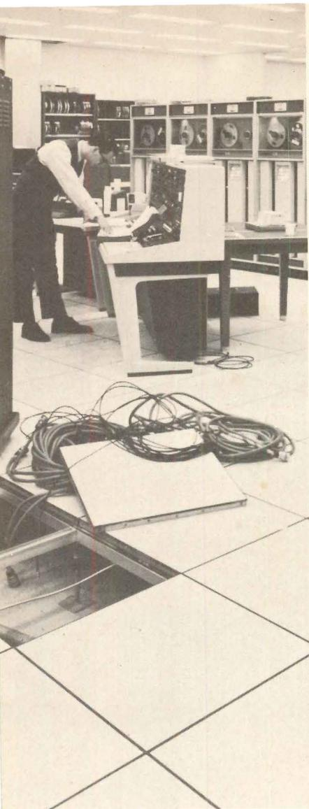
The idea started with computer rooms. Elaflor's vinyl plenum seal combined with Liskey-Aire modular air conditioning units gave highly effective under-floor cooling circulation while panels lifted out easily for instant access to utilities and cabling.
