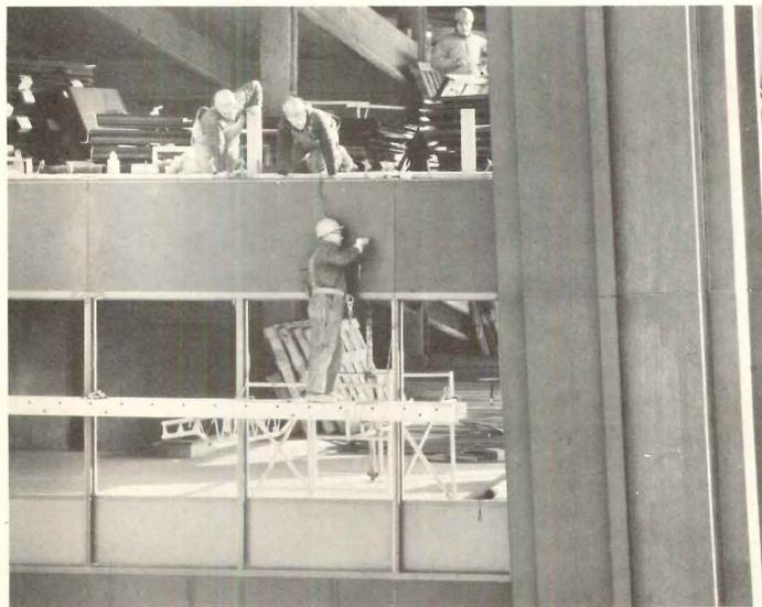
due to the greater exposure and larger size, were insulated with 4-in. urethane. All of the insulation material was attached to the vertical column covers with aluminum insulation nails, applied with a stud welder.
