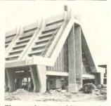
The production of large-scale precast units and their system of assembly at Amberg represent highly advanced industrial building methods. The pilotis and brackets in the top photographs are about to receive the roof ribs shown in place above. Precast columns with x-shaped caps support the lower structure. The triangular shaped end walls of the skylights can be seen in the middle photo.
