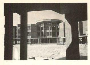
The eight individual buildings of the main school complex will be connected with glazed-in walkways which can be seen in the photo at left. All buildings are built in reinforced concrete poured in situ.
