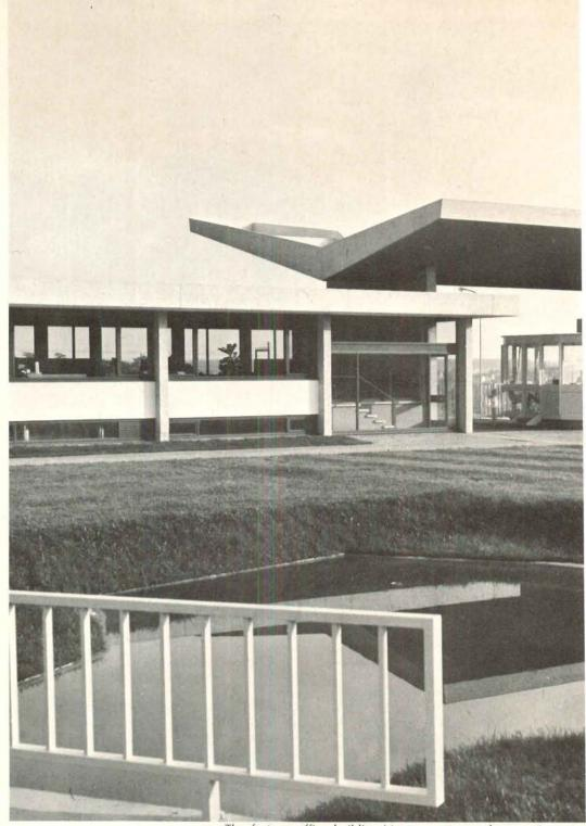
garages, waste silo, and parking area are placed on a site which slopes off to the north and west. The service courtyard is placed on the highest ground to the southeast. The factory is located to the north of this on filled ground. The parking area and bicycle stand, separated by a high retaining wall, slope downhill to the west. The downhill end of the factory exposes a lower production level and service enfor production security, a
