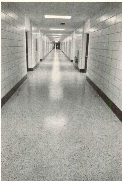
**POURED SEAMLESS FLOORS** / *Florock* is essentially a three step process in which the base coat is poured out, rolled and scattered with chips while still wet. When dry, a liquid polymeric glaze is applied, sanded and re-applied several times. *Florock* floors are said to be easy to clean, weather resistant, not subject to yellowing, durable and able to maintain their luster for years. ■ Crawford Laboratories, Chicago.
