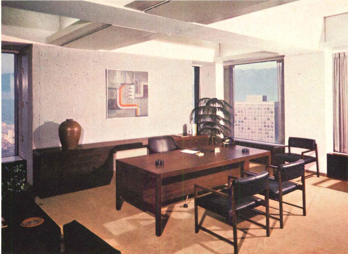
The ceiling grid—structural beams crossed by air-conditioning ducts—is left exposed, economically providing unusual spaciousness for office areas: under beams, height is 8 feet 8 inches; between beams, 11 feet. In the coffer thus produced, 7 feet square, a single light fixture is sus-
