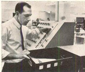
Mail room clerk sends basket to designated floor simply by pushing a button. Each tote box carries up to 32 lbs. of payload . . . the conveyor accepts up to 12 loads a minute.
