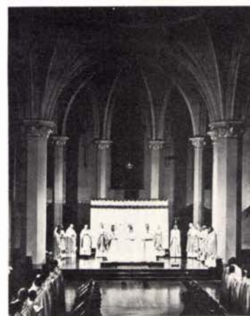
Abbey of Gethsemani , Trappist, Ky., was renovated by William Schickel in collaboration with Jones, Peacock, Garn and Partners, architects, Cincinnati. True structure was revealed through removal of false plaster vaults (above) making the building more compatible with the new liturgy.
