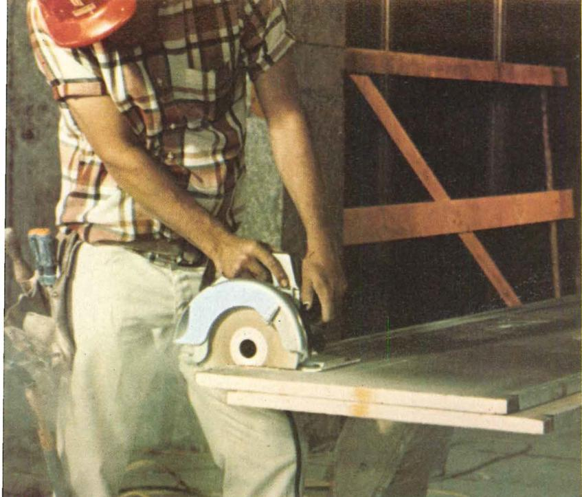
**1** Panel ends are trimmed on-site with conventional equipment. Gold Bond Metaledge Corewall comes in panels 2 inches thick, 2 feet wide and up to 16 feet long.
