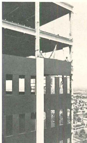
**Martin Tower**, Bethlehem Steel Corporation's new office tower in Bethlehem, has a unique curtain wall of panels fabricated from 3/16-in.-thick steel plate. Pointed tabs projecting upward from the top of a panel are received by openings in the bottom of the panel above. The panels are locked in place and then they are welded at the sides to the building's columns and to angles along the beams.
