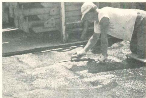
**FLOOR SURFACING** / Latex/cement material is said to withstand loads as great as 18,000 psi. Typical applications include indoor and outdoor loading docks and ramps, and storage areas. ■ Permafex Products Co., Philadelphia.
