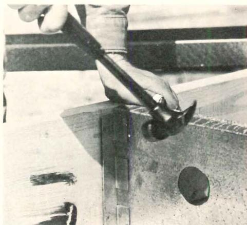
**STEEL FLOOR JOISTS** / End clips nailed to standard band board hold joists in position. Stairway and fireplace openings are formed by heading the joists. Hanger brackets support headers and tail joists. Decking is added and secured by self-tapping screws. ■ Armco Steel Corp., Middletown, Ohio.
