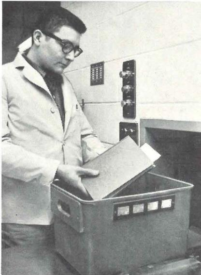
Automatic control is an integral part of a Recordlift System. It employs the magnetic tab principle of conveying encoded digital information—one of the most reliable, economical, maintenance-free systems devised.
