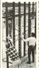
load-bearing panels have been used to replace individual steel members in a recently built apartment complex. Eight different panel sizes are being supplied by the manufacturer; panels include necessary openings for windows, doors, and heating, ventilating and air conditioning equipment. Panels, which can be erected immediately, replace individual studs welded on job site.
