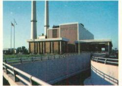
The specifications called for a coating that would last 20 years. That's why the 80 foot-high extruded aluminum louver assemblies on this incinerator plant were factory finished with longlife DURANAR 200 fluoropolymer coatings from PPG.
