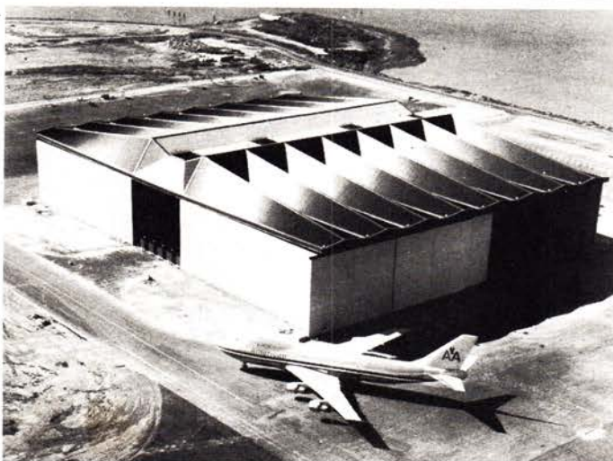
Hangar roof—a new concept—could be left exposed.
