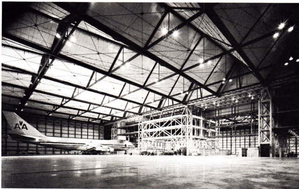
Hangar roof—a new concept—could be left exposed.
