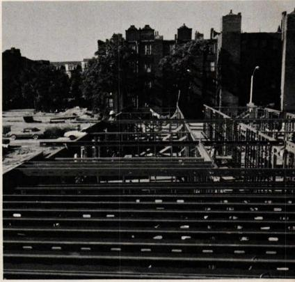
Viviendas La Victoria is a Boston housing project by John Sharratt Associates. There are 151,000 sq. ft. of steel framing in the wall areas; 83,000 sq. ft. of floor joist framing and 20,000 sq. ft. of specially-designed fabricated steel trusses in the roof framing systems.
