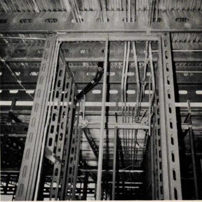
The cavity created by steel framing allows for continuous insulation of the walls. This was important to Architect Elam Denham in designing a unique hospital/nursing home in Bella Vista, Ark. State law requires nursing homes be heated as high as  $80^{\circ}$ . Steel frame structures insulate well.
