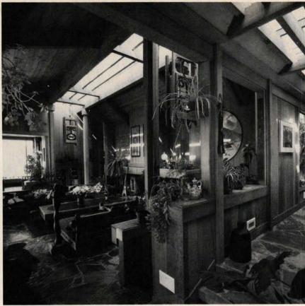
The range of primary finish materials inside is controlled: cedar siding for paneling, waxed slate for some floors, pine boards for others, plastic for skylights. Outside, the house is clad in random width cedar boards laid up vertically and the roof is covered in concrete shingle.
