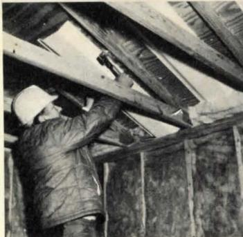
**ROOF VENT** / Designed to provide necessary air ventilation from soffit to attic, 48-in.-long *Proper Vents* are stapled to the underside of roof sheathing at the cornice and plate line. Each vent provides a 16-sq.-in. air space to control attic moisture and prevent ice buildup and damming on the roof. ■ WayneRoy, Inc., Minneapolis, Minn.
