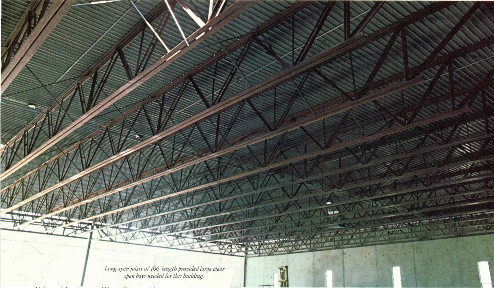
*Long-span joists of 106' length provided large clear span bays needed for this building.*
