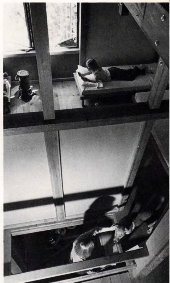
To ease the erection process, Kindorf framed out the floors in doubled 2x6s, bolted in place, and the roof in 2x8s, also paired. Floor planking is white fir, roof is galvanized sheet.
