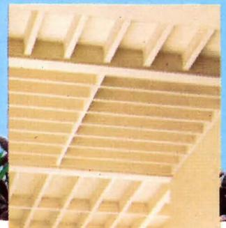
One-way joist floor system was used throughout. Eye pleasing ribs are in an alternating pattern perpendicular or parallel to the shear walls and spandrel beams.
