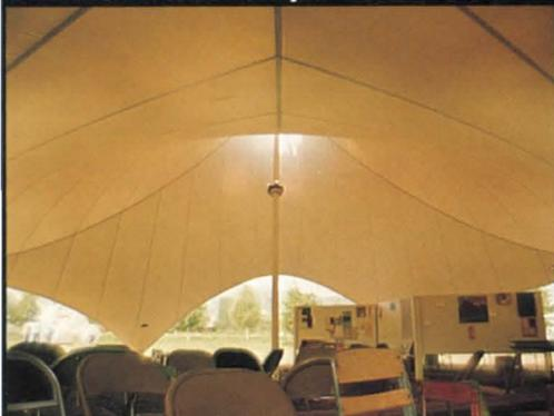
The logic of this tensioned membrane structure is as exciting as its appearance. A canopy over a school yard play area, it provides shelter for outdoor activities in almost any weather. The attractive "upside-down" design allows rain water run-off through the support columns.
