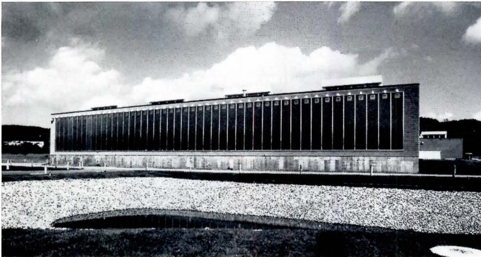
The Trombe wall for a warehouse addition at Famolare headquarters in Vermont is 184 ft long and is oriented 10 degrees east of due south. The warehouse is windowless except for 16 roof monitors. The pond in the foreground of the above photo is an absorption basin for rainwater drainage from roof and paving. The wall is expected to contribute 38 per cent of the building's
