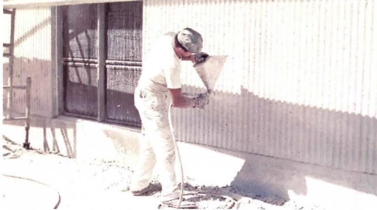
To begin with 40,000 tie-rod holes were patched with THORITE, the nonslump, nonshrink patching mortar before all concrete surfaces, inside and out, of this library were sprayed with two coats of THOROSEAL PLASTER MIX, cement-base, waterproof coating, PLUS ACRYL 60, adhesive bonding agent. The primary purpose of this finish not only waterproofs and preserves these surfaces for as long as they stand, but maintains the architectural detailing with a beautiful, uniform white texture over all.
