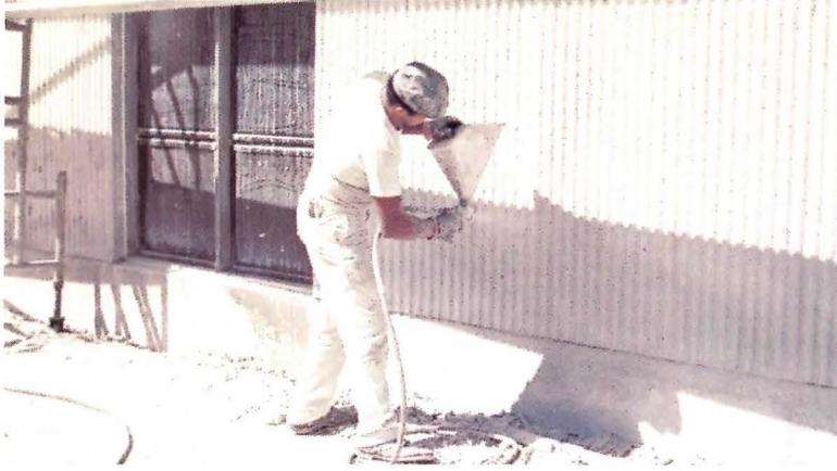
To begin with 40,000 tie-rod holes were patched with THORITE, the nonslump, nonshrink patching mortar before all concrete surfaces, inside and out, of this library were sprayed with two coats of THOROSEAL PLASTER MIX, cement-base, waterproof coating, PLUS ACRYL 60, adhesive bonding agent. The primary purpose of this finish not only waterproofs and preserves these surfaces for as long as they stand, but maintains the architectural detailing with a beautiful, uniform white texture over all.
